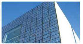
The façade of this building has integrated PV panels built into it. Photo: www.solarcentury.com
