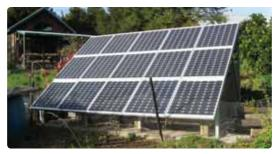
This photovoltaic array uses an inclined frame mounted on the ground. Photo: Genkit Nelson Ltd.
