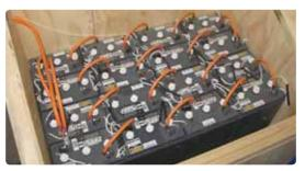
The batteries for this SAPS are well protected and secured in this box, preventing unauthorised access. Photo: SEANZ
