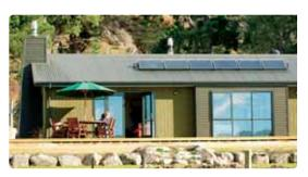
A solar water heating system installed with a stand alone power system. The house does not have a connection to the electricity network.
