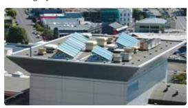
A commercial-scale solar water heating array installed on the Sky City building in Auckland.
