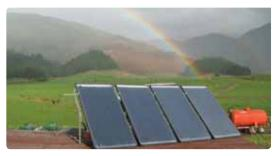
Frame-mounted solar water heating collector panels installed on a dairy shed.
