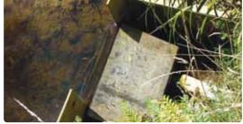
Another example of an intake structure. The stream flows over the metal screen, which prevents leaves or debris from entering the white plastic penstock.
