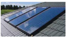
Frame-mounted flat plate collector panels.
