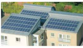
Photovoltaics are becoming increasingly common in grid-connected systems in urban environments. Photo: www.solarcentury.com
