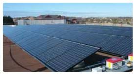
Frame mounted grid-connected PV system. Photo: www.solarcentury.com
