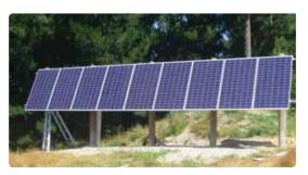
A ground mounted photovoltaic array. Photo: www.powersmartsolar.com
