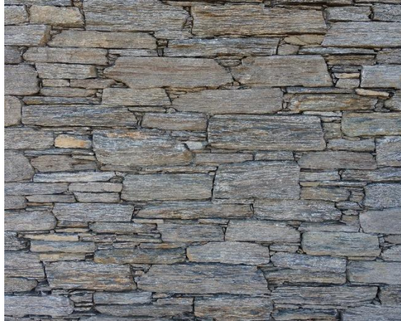
Fig 1: Dry-stacked schist
