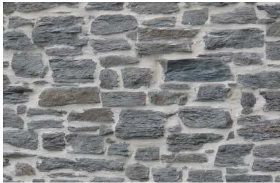
Fig 2: Bagged Schist
