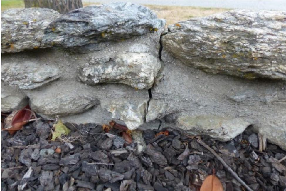
*Figure 7: Example of cracks in the front wall*
