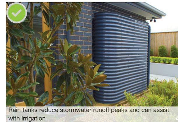
Rain tanks reduce stormwater runoff peaks and can assist with irrigation
