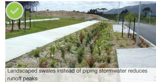
Landscaped swales instead of piping stormwater reduces runoff peaks
