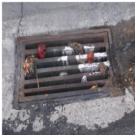
Figure 3: Evidence of paint disposed down the stormwater system
