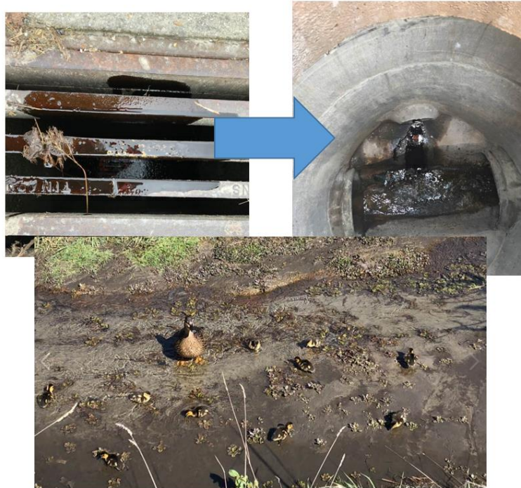
Figure 2: Used motor oil poured into the stormwater system
