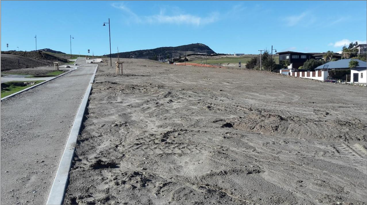
Figure 4: Unstabilised slope with rill erosion.
