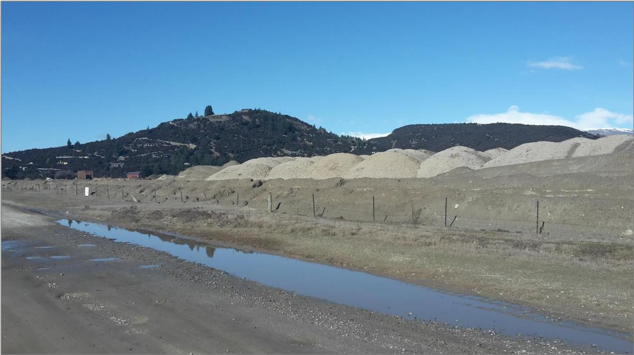
Figure 1: Topsoil stockpiles with no sediment control
