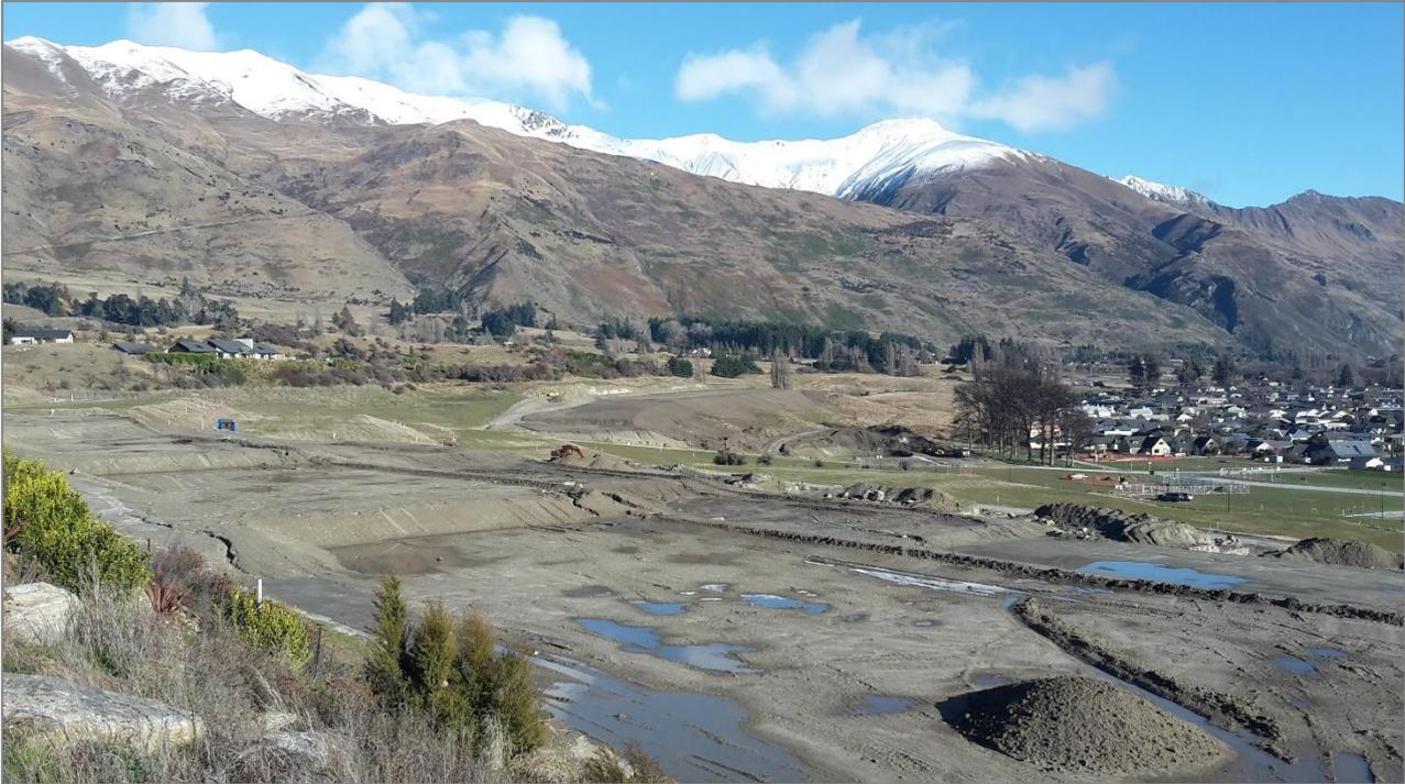
Figure 6: Open earthworks areas with no clear staging or progressive stabilisation
