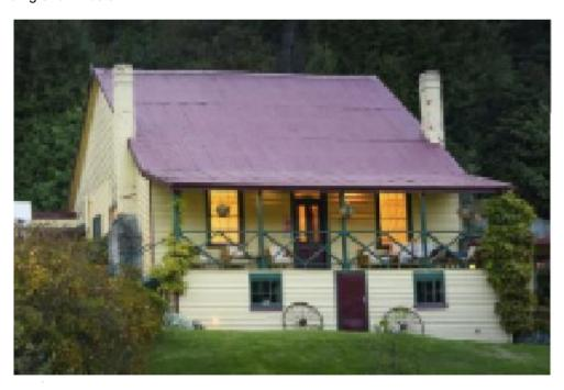
From my review of the photographs you provided the single level building structure comprises light weight timber framing for floors, walls and roof and there are two tall brick chimneys to each of the gable ends. Timber framed structures of this type are not typically earthquake prone but the two chimneys would be unless strengthened.
