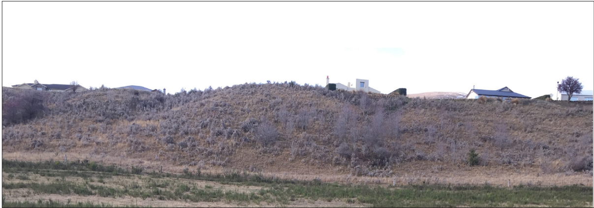
Photograph of the existing escarpment, which was sprayed in March 2014
