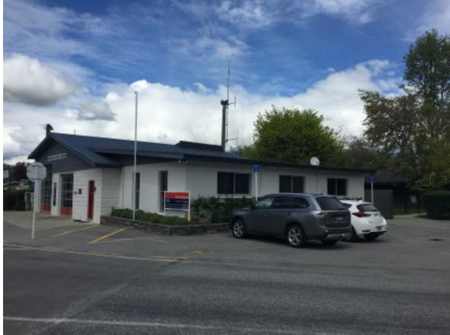
Photo 2: Arrowtown Fire Station (from Wiltshire Street looking south)
