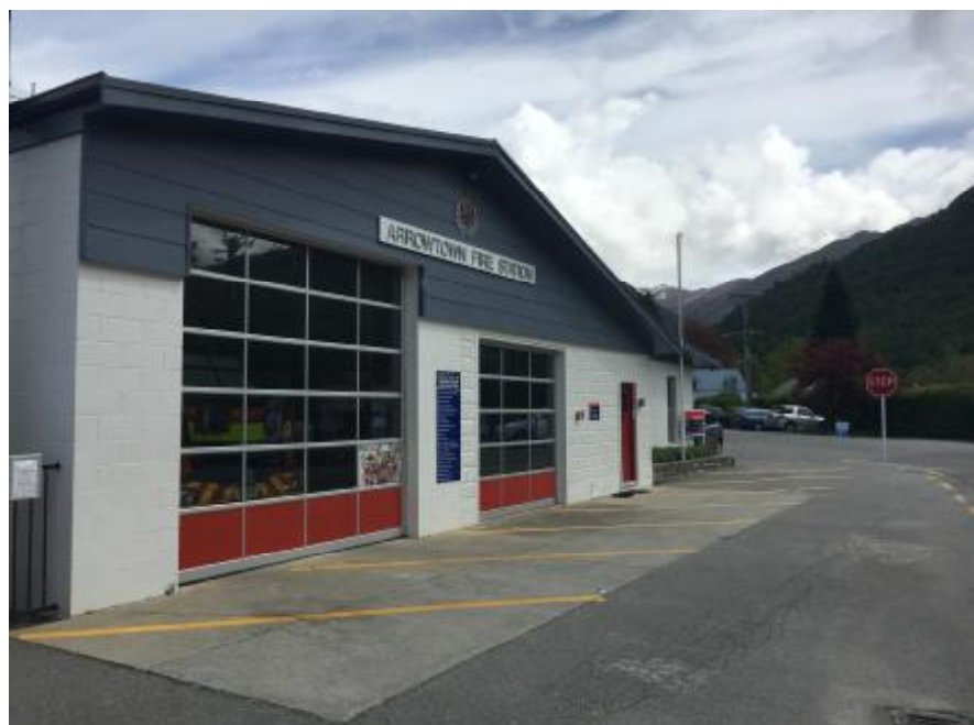
Photo 1: Arrowtown Fire Station (from Hertford Street looking north west towards Wiltshire Street)
