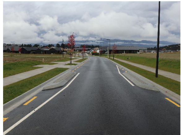
Photo F: Lammermoor Street Road localised narrowing
