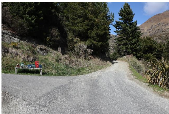
Figure 7-5: Narrow entry into the curve on Atley lane section (southbound). Note poor intervisibility due to cutting either side.
