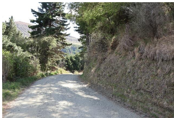
Figure 7-6: : Narrow entry into the curve on Atley lane section (westbound). Note poor intervisibility due to cutting either side
