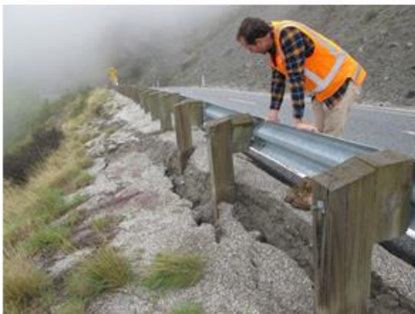
Figure 7. Cracking and settlement at the road shoulder at site 3.
