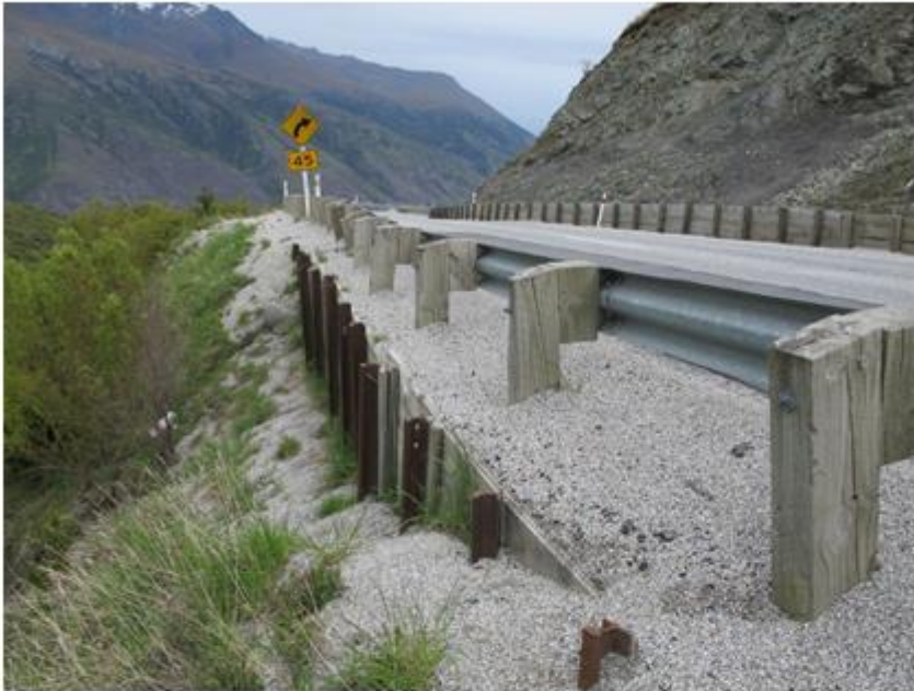
Figure 13. Site 6 driven rail iron wall
