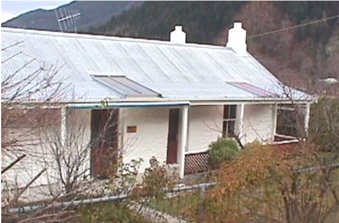
Thompson House 66 Hallenstein Street, Queenstown
