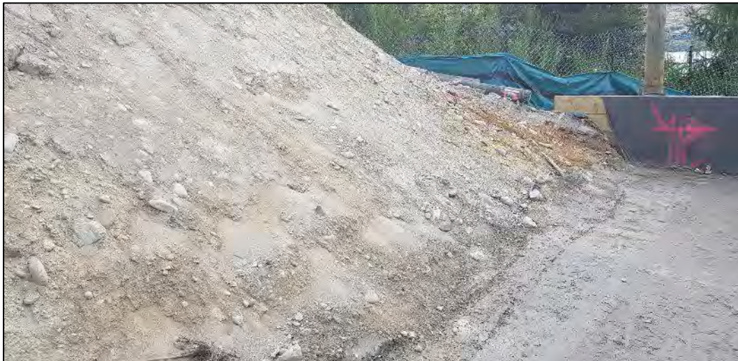
Photo 2: Soil batter trimmed down to expose natural ground.
