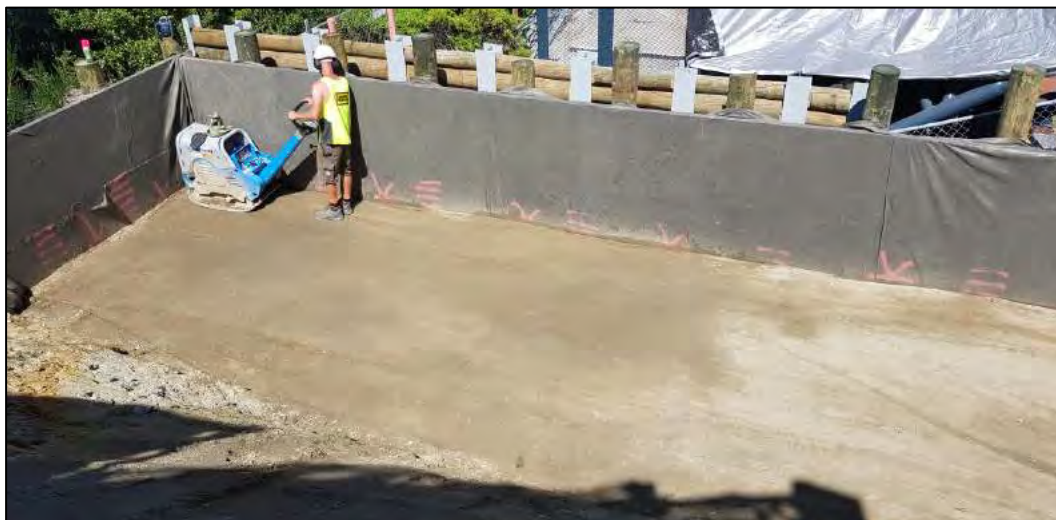
Photo 1: Looking south across the fill placed behind the retaining wall.
