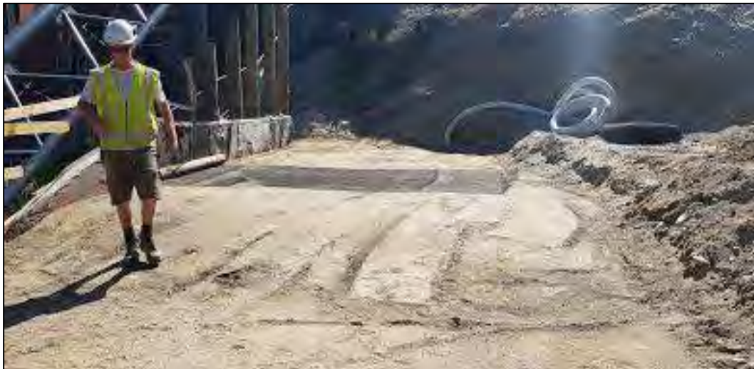
Photo 2: Looking north across the lower pad following placement of an additional 400 mm of fill.
