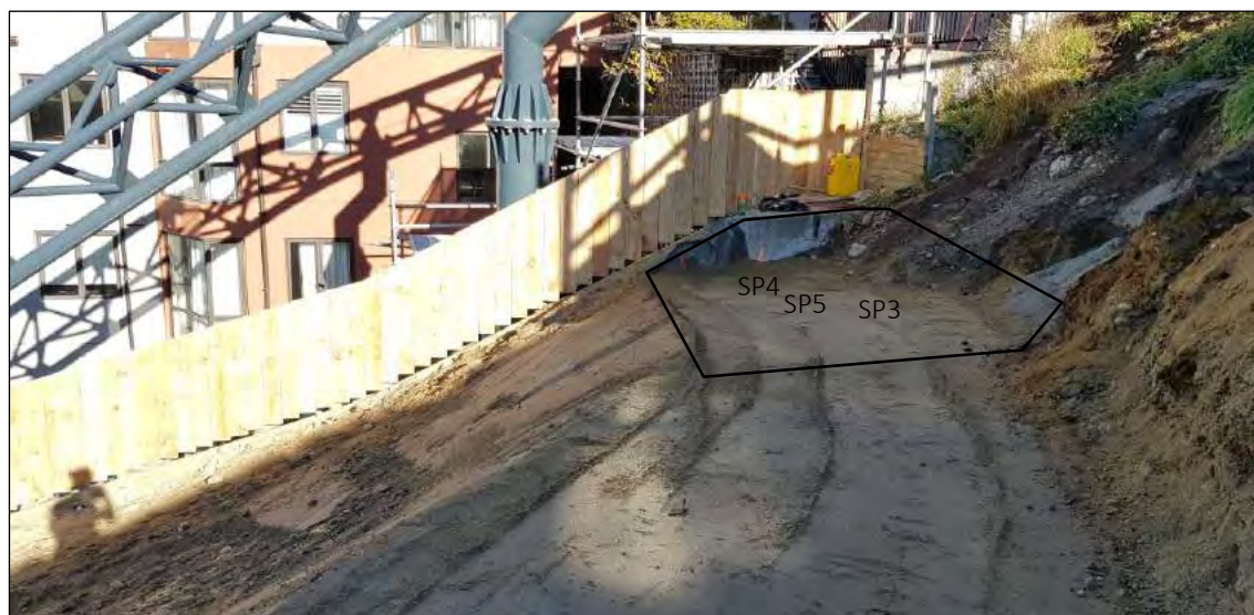
Photo 2: 2.0 m fill testing. Test locations indicated on the photo. Small area of fill remaining.
