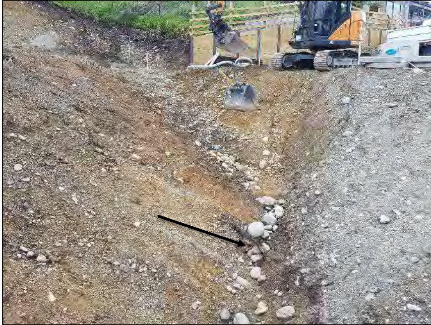
Photo 1: Looking north-west across the undercut gully located along the access road. Subsoil drainage to be placed along the base of the gully.
