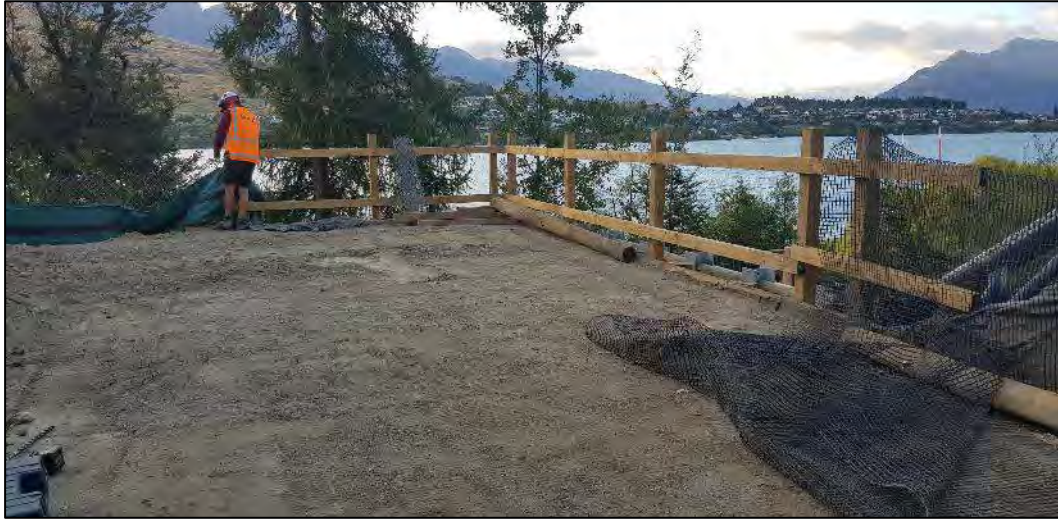
Photo 1: Looking south across the fill area located behind the retaining wall. The southern end of the fill is at finished level whereas the northern end will be further backfilled at stages.
