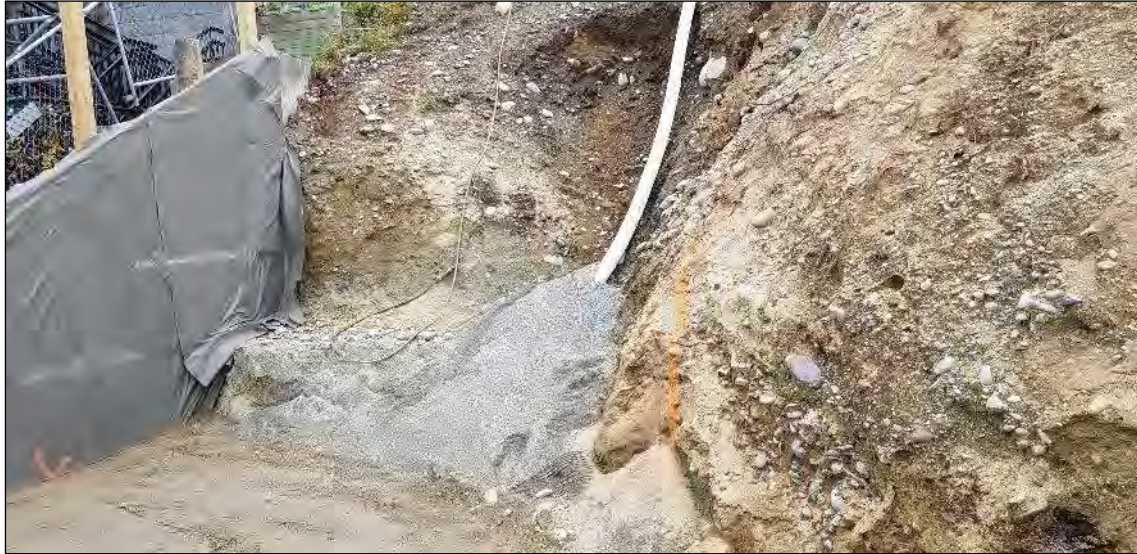
Photo 1: A drain coil is placed horizontally along the edge of the fill surrounded by bedding sand. The drain coil is connected to the drain coil running along the eastern edge of the fill (indicated on photo).
