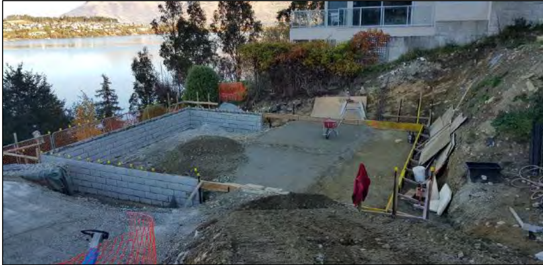
Photo 1: Looking across the building footprint of Unit 6. The western portion of the building footprint is founded on natural ground.
