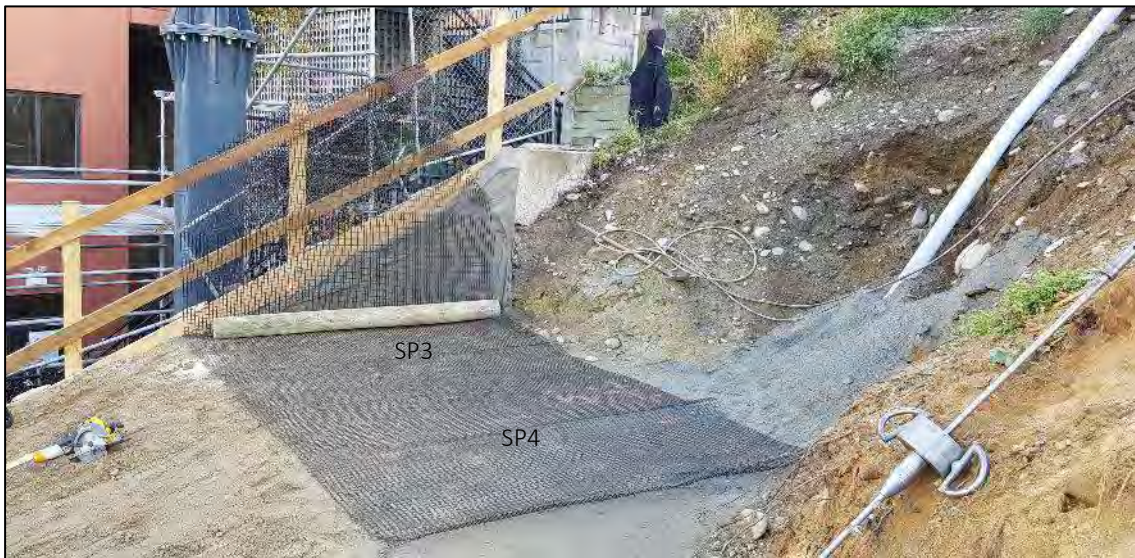
Photo 2: Fill testing following placement of additional 500 mm of fill. Test locations indicated on the photo.
