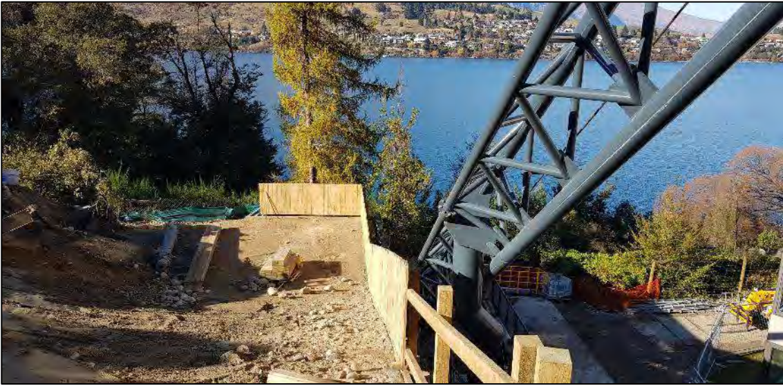
Photo 1: Looking south-east across the fill placed behind the timber retaining wall.
