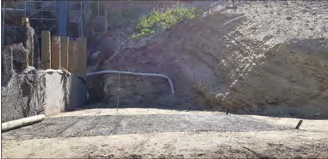
Photo 1: Looking north across the lower pad. 4.0 m of fill placed in total.
