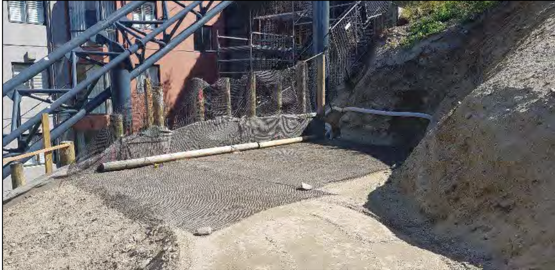
Photo 2: Looking north-west across the lower pad. 4.5 m of fill placed in total.
