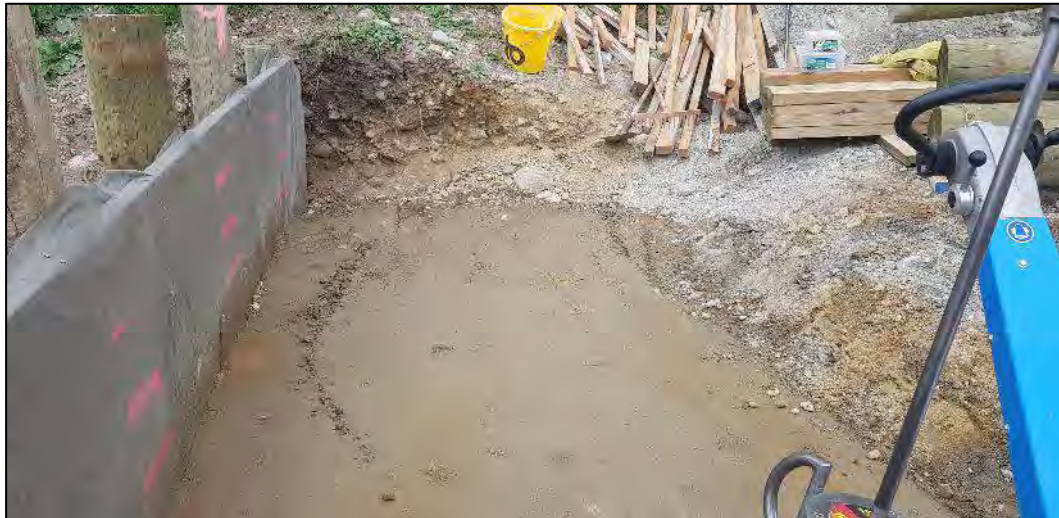
Photo 1: Looking north across the fill placed along the timber retaining wall for the access road.
