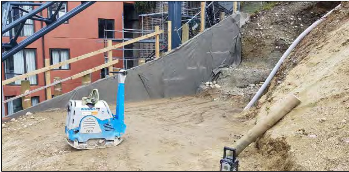
Photo 1: The northern portion of the fill did not achieve required compaction and had a high water content.
