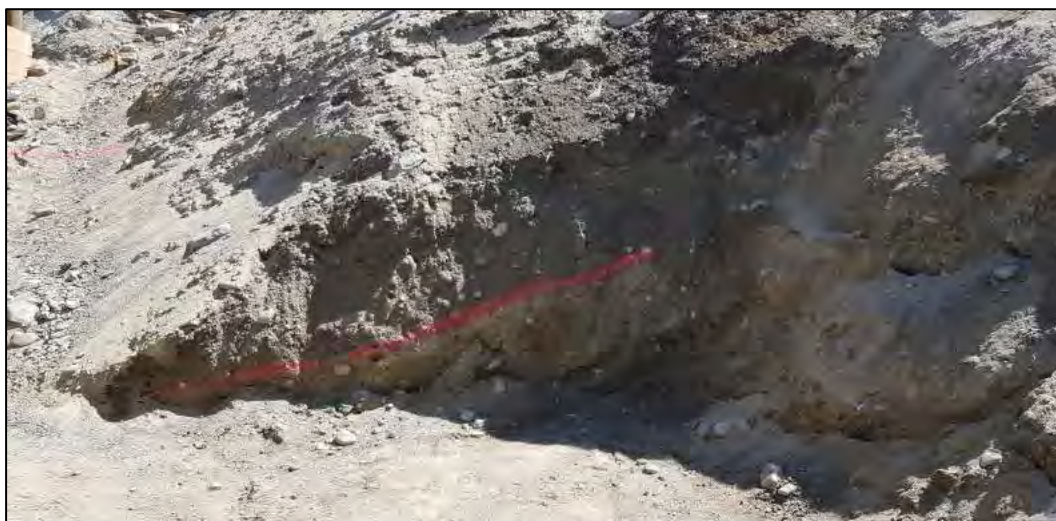
Photo 2: The boundary between natural ground and fill had been marked out for the soil batter located upslope from the engineered fill.
