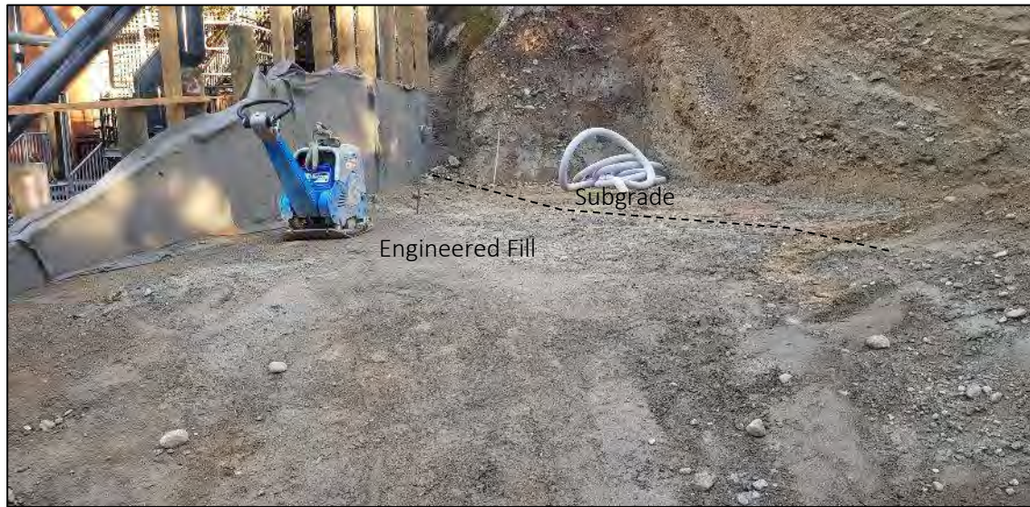
Photo 1: Looking north across the lower pad. 3.5 m of fill placed in total with natural subgrade exposed at the northern end.
