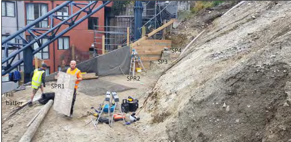
Photo 1: Looking north-west across the lower pad. ~1.0 m of fill placed in total. The fill will be placed up to/just below the top of the timber retaining wall along the western boundary.
