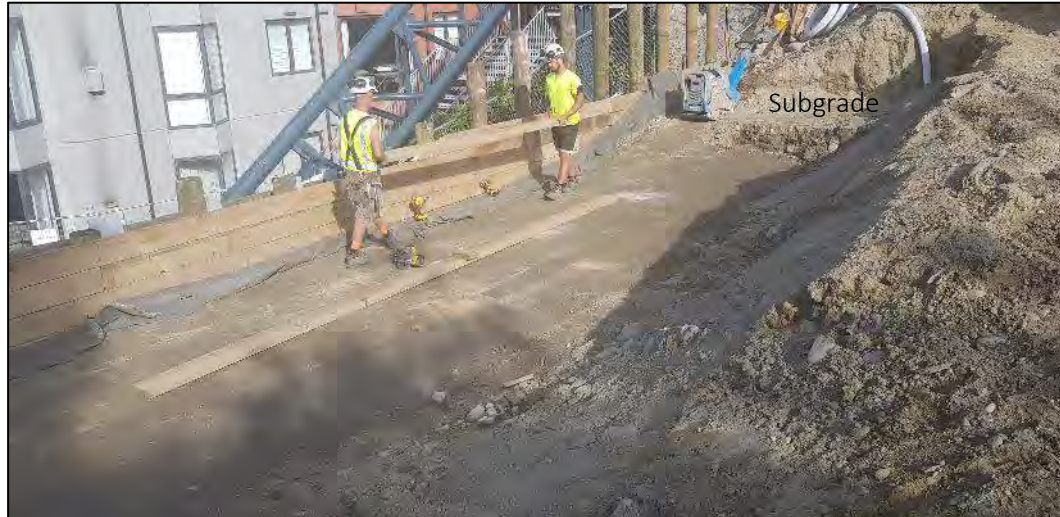
Photo 1: Looking north-west across the fill placed along behind the retaining wall and the subgrade exposed at the northern end.
