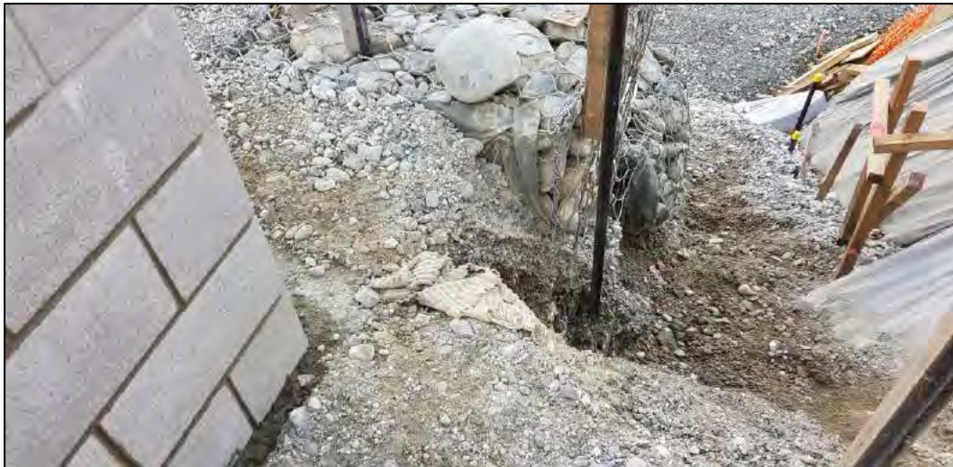
Photo 2: Looking at the southern corner of Unit 6 and the end of the gabion wall. The fill along the end had started eroding due to rainfall.
