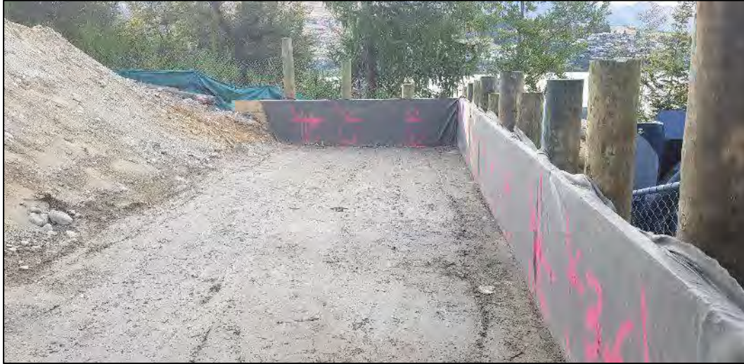
Photo 1: Looking south across the fill placed behind the retaining wall, 1500 mm.
