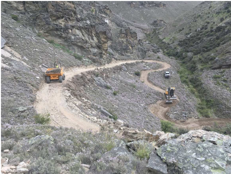
Photo 2: Almost completed trail near Halfway Hut, Lake Dunstan Trail. Note the revegetated fill batter slopes
