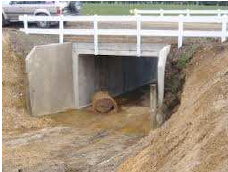
Figure 2: Typical road underpass for stock or cyclists
