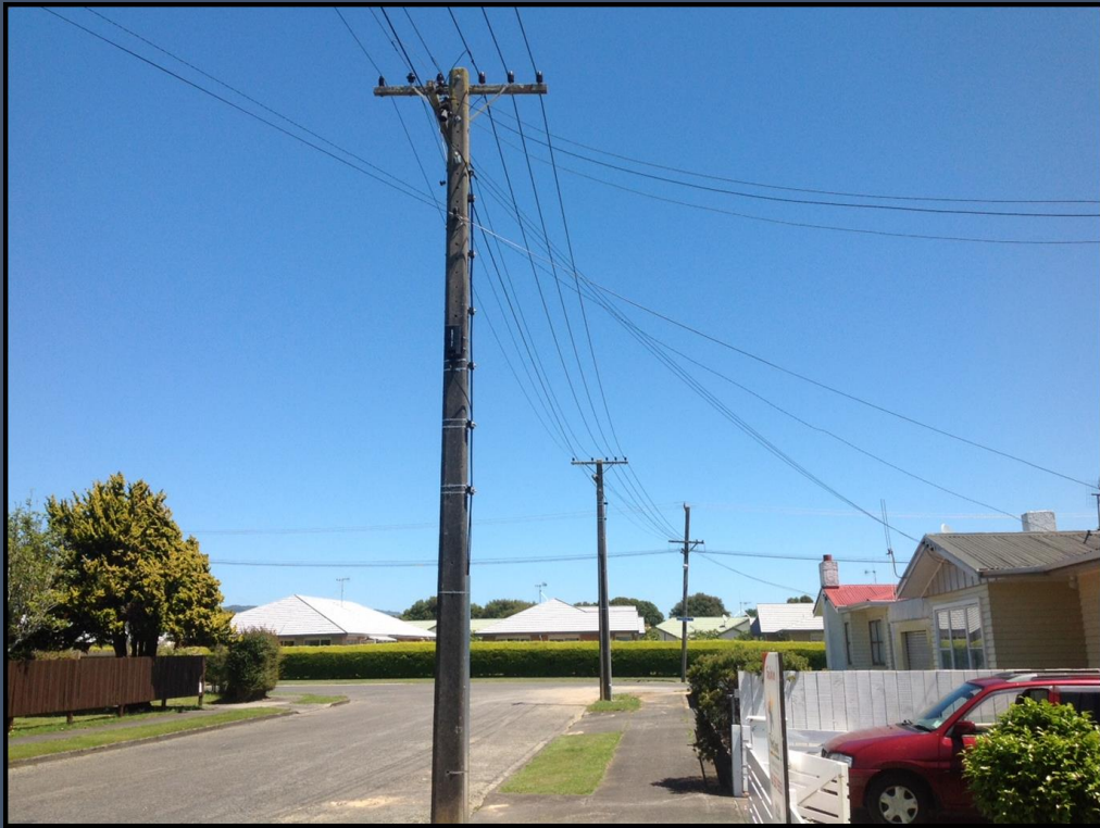
UFB Deployment – Levin (on electricity poles)
