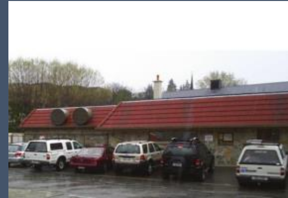
Queenstown Telephone Exchange & Microwave Station
