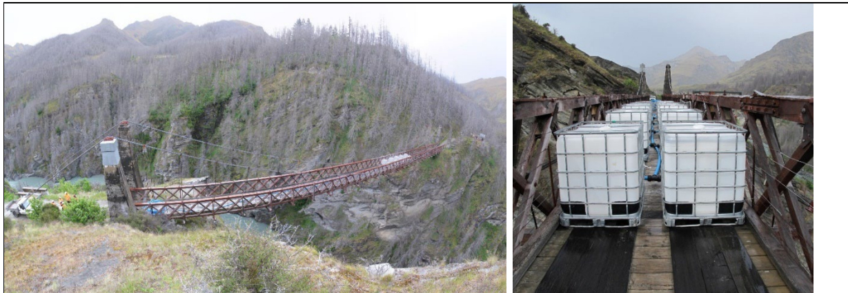
Figure 10. 2021 load testing arrangement
