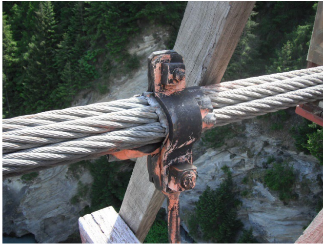
Figure 31. Top section of hanger
