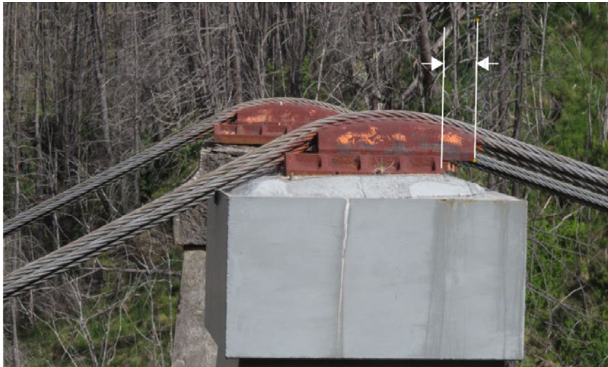
Figure 6. Displacement of the Stoney Roller bearings toward the span on the TL
