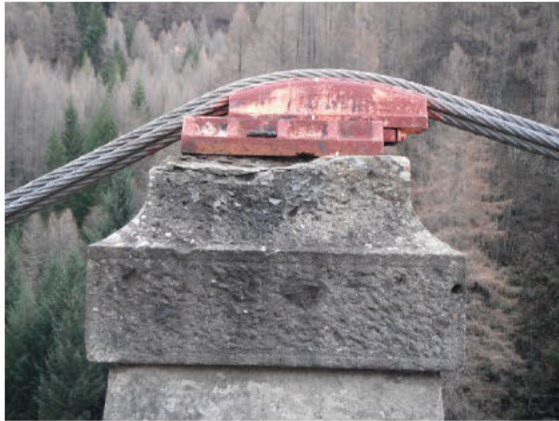
Figure 5. Displaced Stoney Roller bearings on both towers on the TL side 2013. The movement indicates possible relaxation of the TL cable anchorages and introduces eccentric loading onto the top of the tower.
