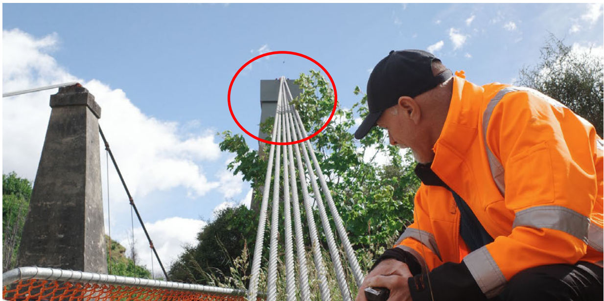
Figure 11. Bundling of the cables over the tower and span
