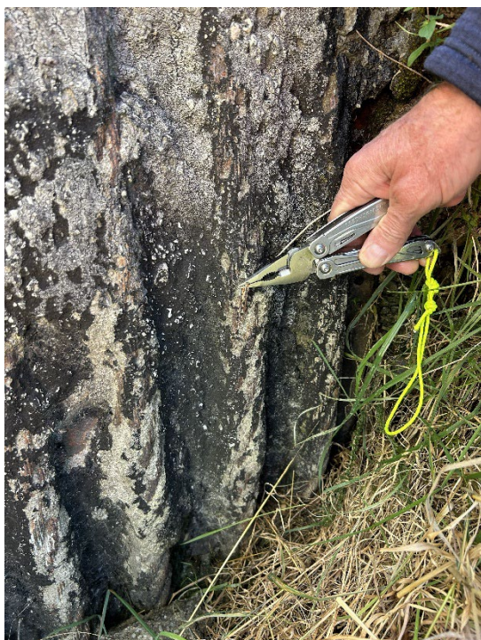
Figure 5. True Right, US cable- insignificant corrosion and no broken wires located
