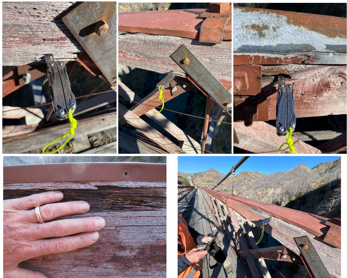
Figure 37. decay in the top chord of the trusses and steel plates to locate the truss cross bracing
