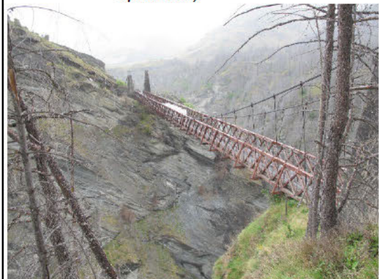
Figure 30. TL abutment and bluff with adverse schistosity (looking upstream)
