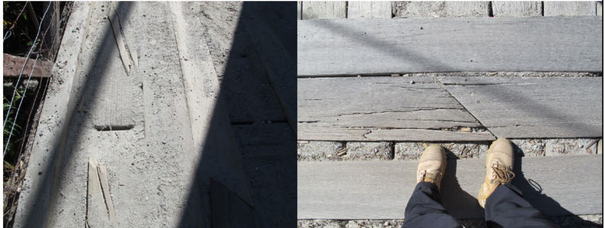
Figure 40. Degraded and split running planks on the TR end of the bridge
