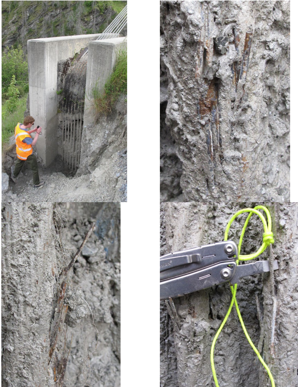
Figure 9. Cable damage on DS TL cables
