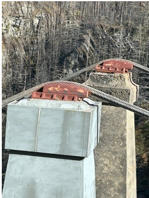
Figure 24. TL towers and displaced bearings. Decay of downstream TL basalt capping block visible. Steel jacket installed in 2013.
