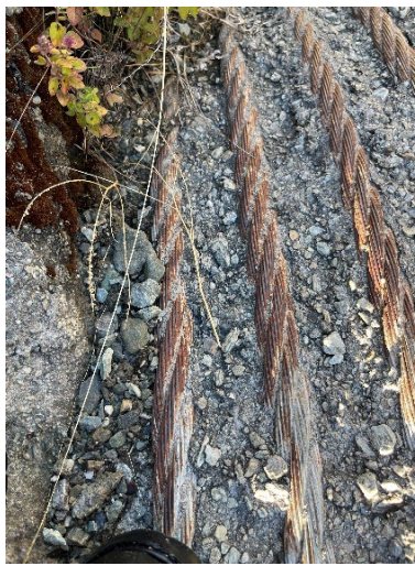
Figure 22. TL downstream surface corrosion of cables
