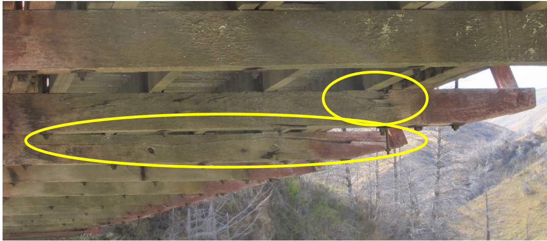
Figure 33. typical damaged transoms (these have been replaced since this photo)
