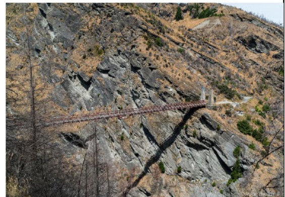
Figure 30. TL abutment and bluff with adverse schistosity (looking upstream)
