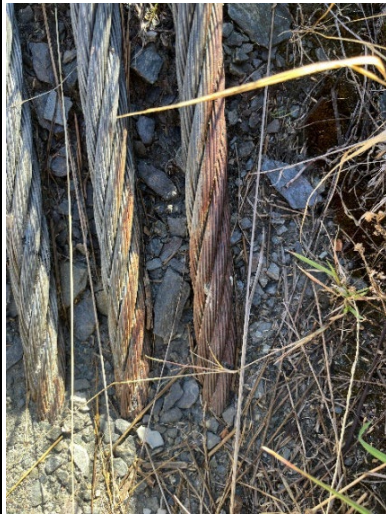
Figure 21. TL upstream surface corrosion of cables
