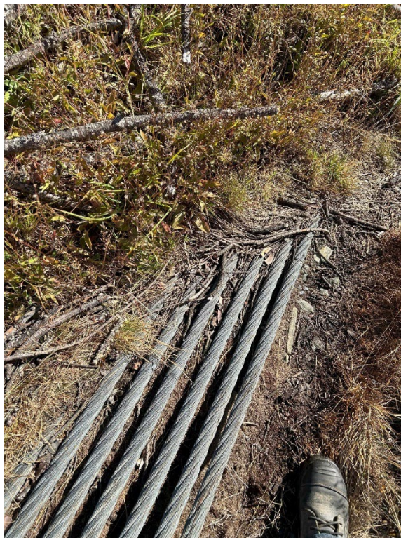
Figure 16. Cables on TR entering the ground with only galvanising of the cables for corrosion protection. No significant corrosion was observed in this location
