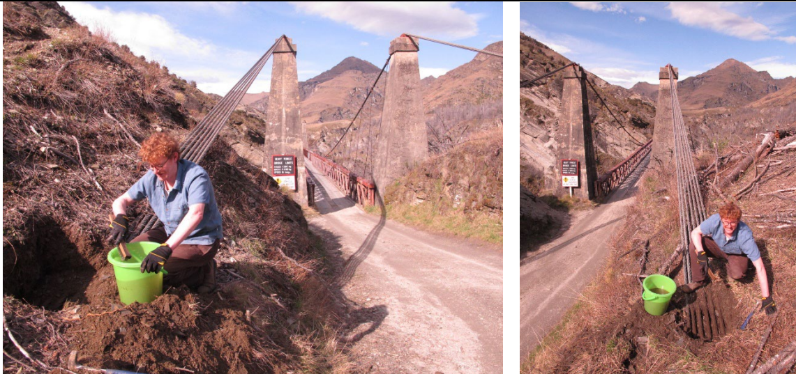
Figure 3. Excavation and cable cleaning on the True Right, Upstream and Downstream sides
