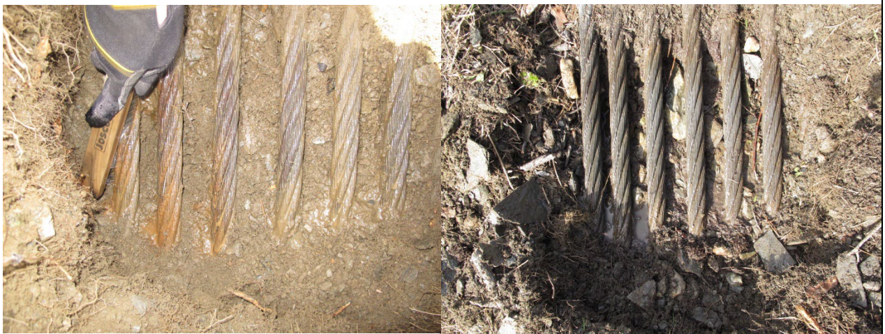
Figure 5. True Right, US cable- insignificant corrosion and no broken wires located
