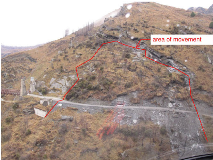
Figure 5. Unstable area showing its proximity to the TL anchorages
