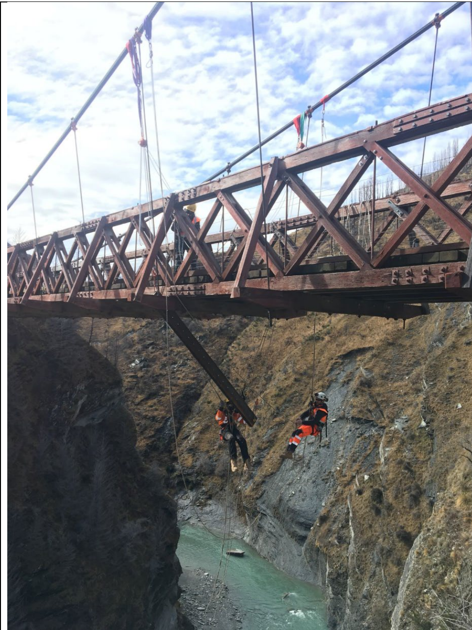
Figure 36. bolting channel section to strengthen a transom in 2019
