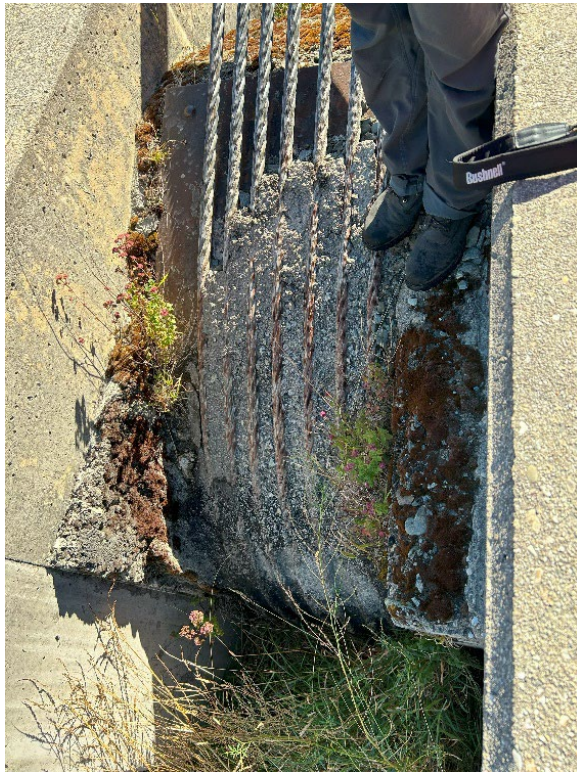
Figure 18. Saddle at TL downstream anchorages where the cables change direction into the anchorage shaft. Note rust on cables
