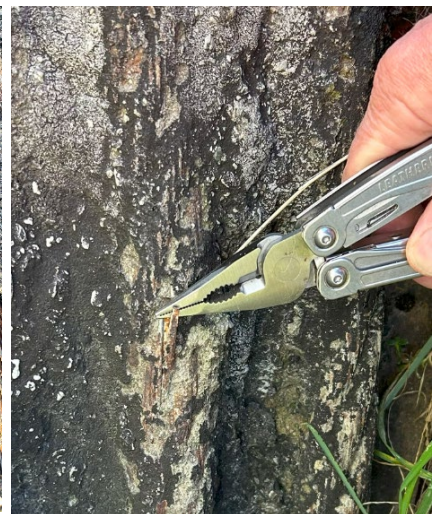
Figure 20. TL Downstream broken strands
