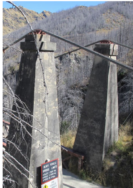
Figure 25. TR towers – these TR do not have stone capping blocks although historical photographs suggest that all four towers originally had basalt capping blocks.
