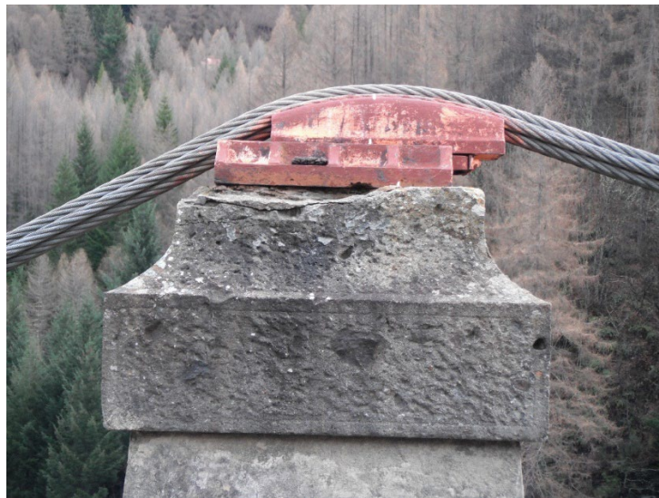
Figure 23. Decay of the TL downstream tower basalt cap and displacement of the bearing
