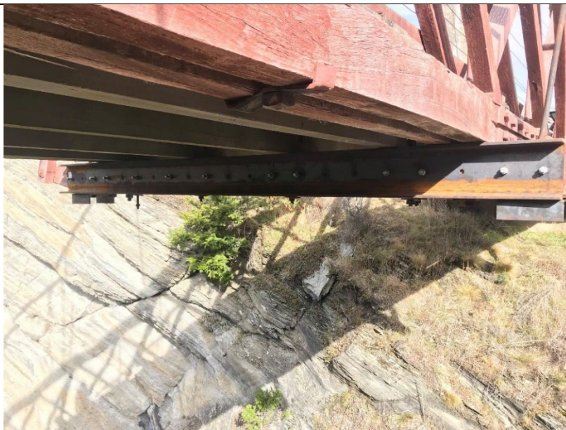
Figure 34. Transoms supplemented with steel channels
