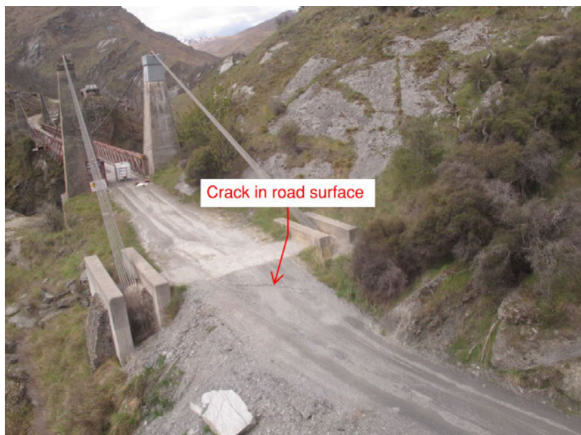
Figure 4. Crack in road surface immediately adjacent to cable anchorages on the TL taken in November 2025.
