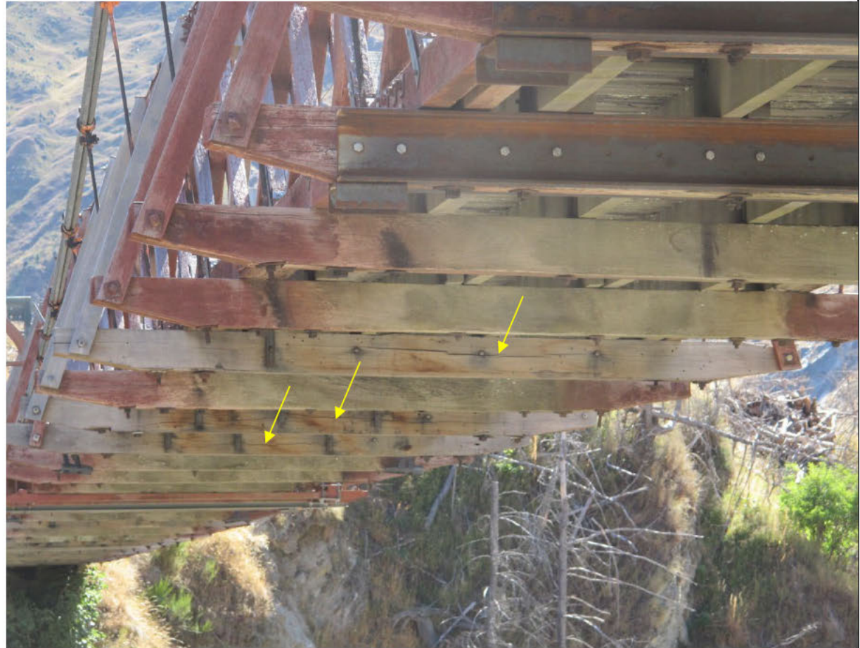
Figure 35. Three timber transoms, replaced within the last four years, identified by the new steel angles to the stringer beams above, which have longitudinal cracking, probably due to drying shrinkage since placement
