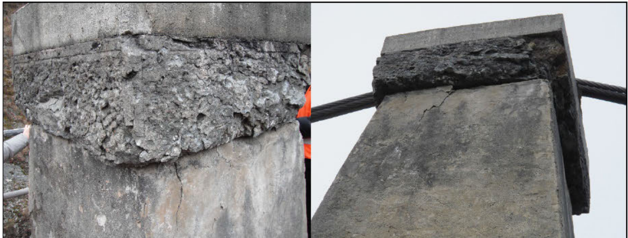
Figure 6. TL upstream tower capping block deterioration and cracking in the tower in 2013 prior to repair of the tower
