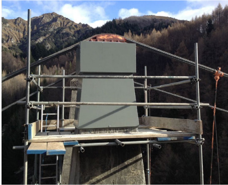
Figure 7 the steel jacket grouted around the capping block and top of the TL upstream tower where cracking of the top of the tower was occurring
