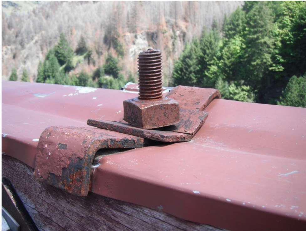
Figure 38. local buckling in truss flashing which may indicate decay of the timber below
