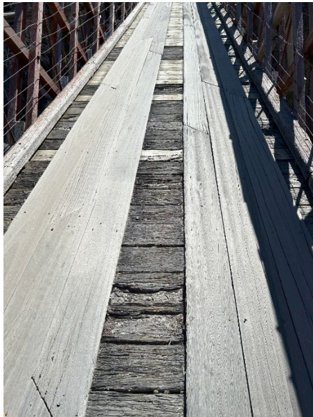
Figure 39. bridge deck consisting of both pine and hardwood planks
