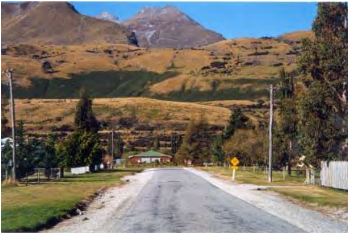
Photos. Narrow carriageway, wide grass verges, no kerb and channel –features in keeping with rural context - Islay Street
