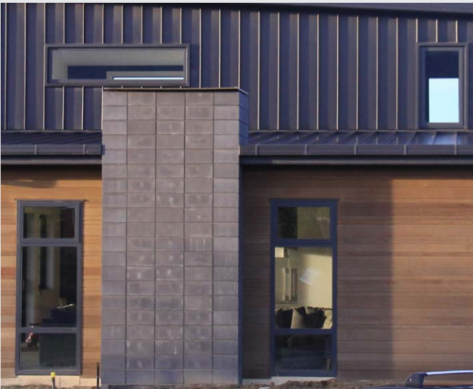
Stack bond masonry block
