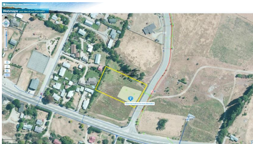
Figure 1 – Subject Site and Existing Services (Storm Water Soakage Basin) Shown Green. Source – QLDC Website 05.03.15
