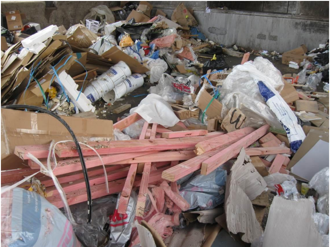
Reusable framing timber in trailer load of construction waste
