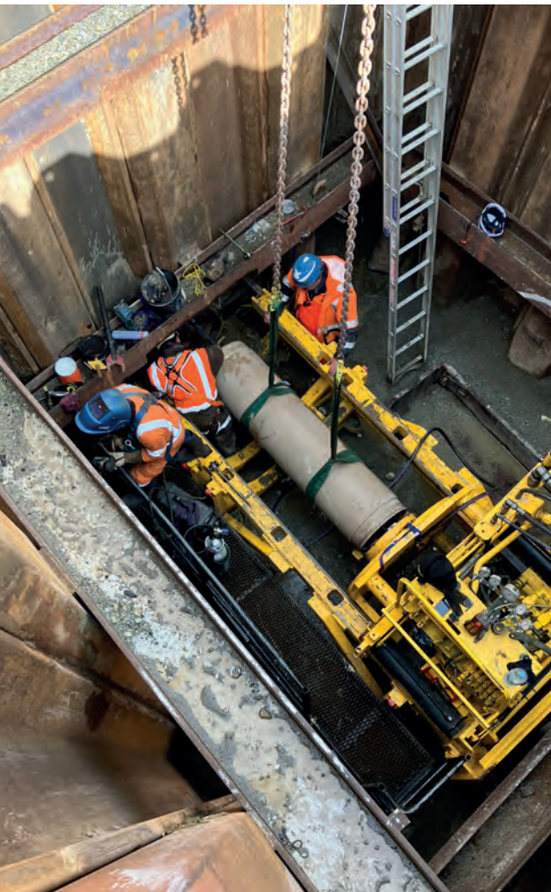
Pipe installation between access pits.
