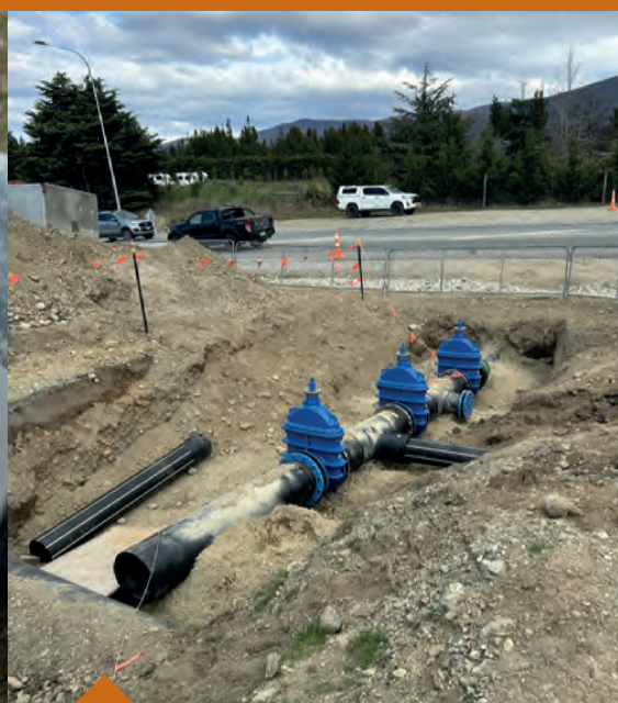
Final major section of 315mm diameter pipe connected to the manifold at Mount Iron Roundabout.
