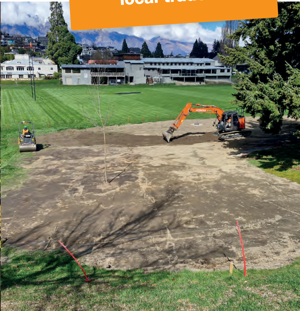
Final touches being applied to the Recreation Ground, including topsoil placement and grass seeding.
