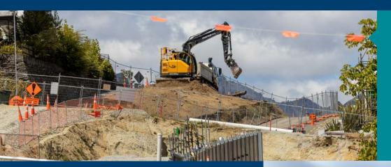
A digger works on constructing the new link between Melbourne and Henry Streets. In the foreground you can see the large steel sheets which have been dug into the ground to help form the new road.
