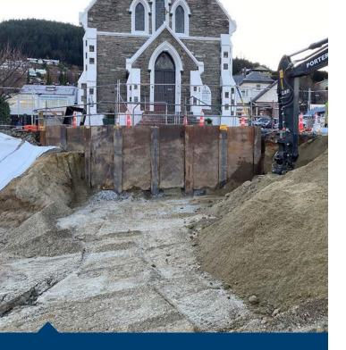
A steel wall is being built in front of the St Joseph's church and school, ahead of the main retaining wall construction.
