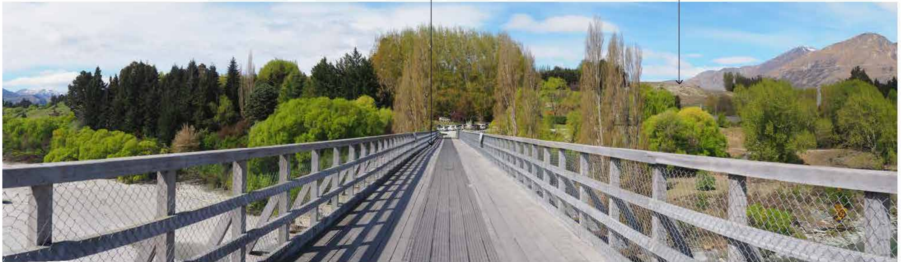
Viewpoint Photograph 9: From Shotover Bridge (looking east)
