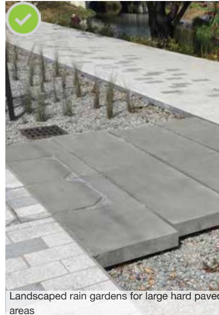
Landscaped swales instead of piping stormwater reduces runoff peaks
