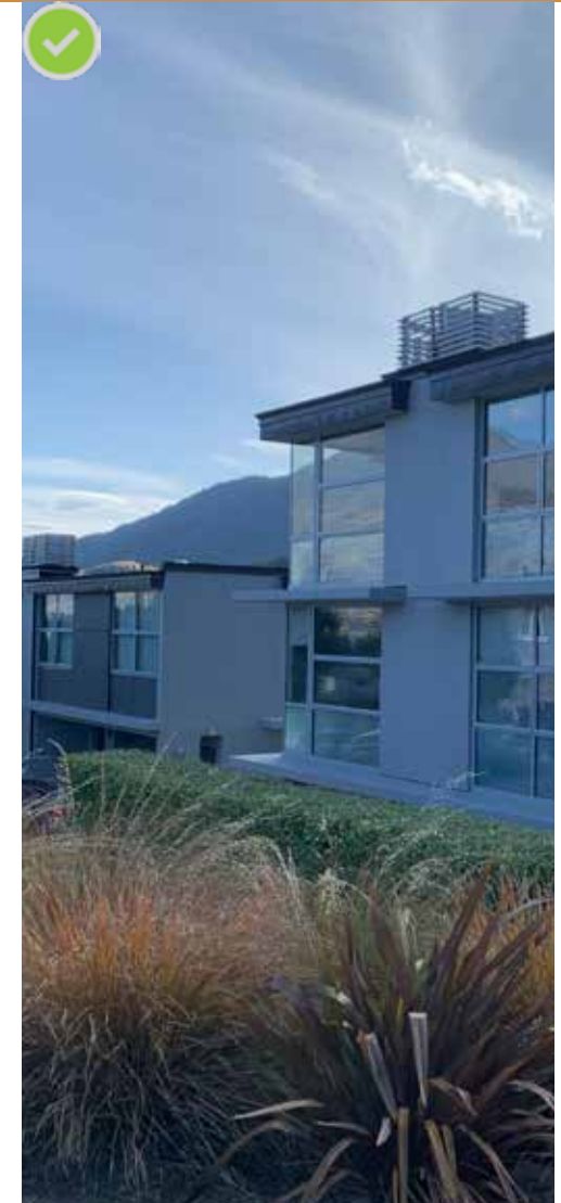
Flat roofs can allow views from buildings behind to be maintained.
