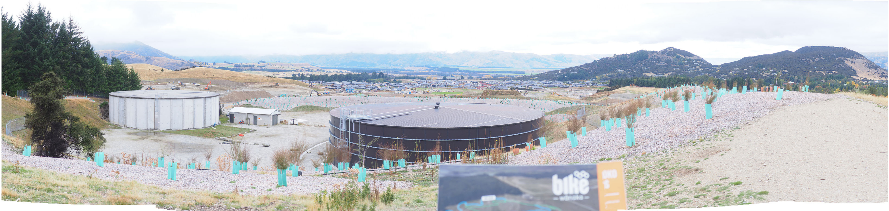
Viewpoint 8. Located at the summit of the Kirimoko bike trail, adjacent to the water tanks, look northeast on the Site boundary.
