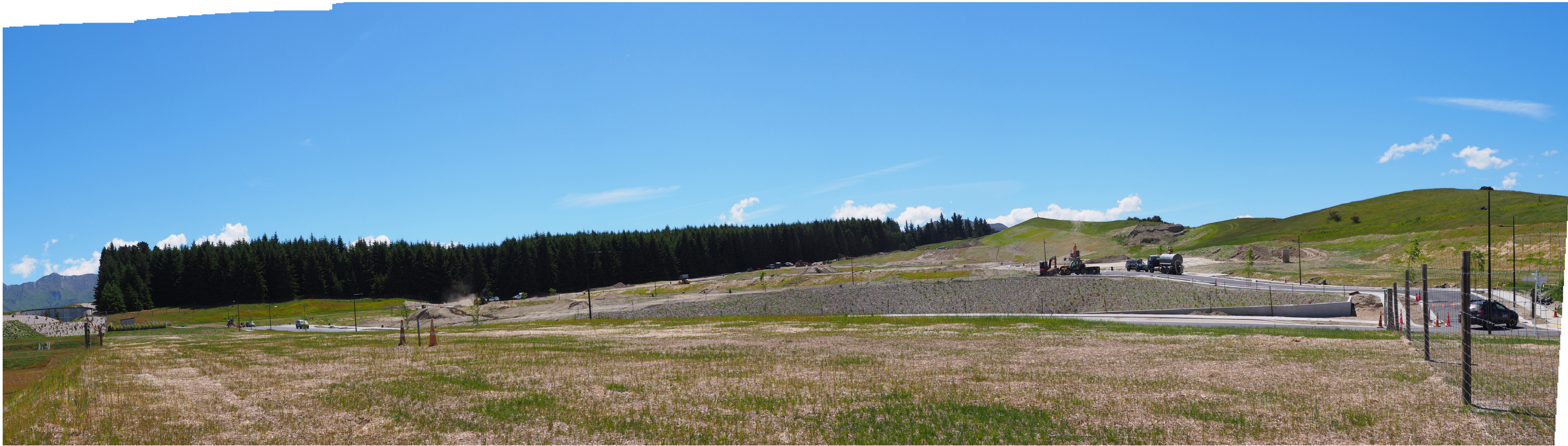
Viewpoint 10: Located within the Site, at the end of Lammermoor St, Northlake looking northwest towards the proposed extension area of the Site at a distance of 150m
