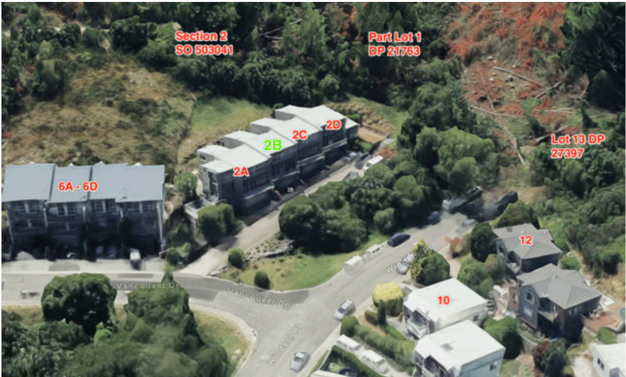
Figure 6 – The Subject Site & Adjacent Land (3D View)
