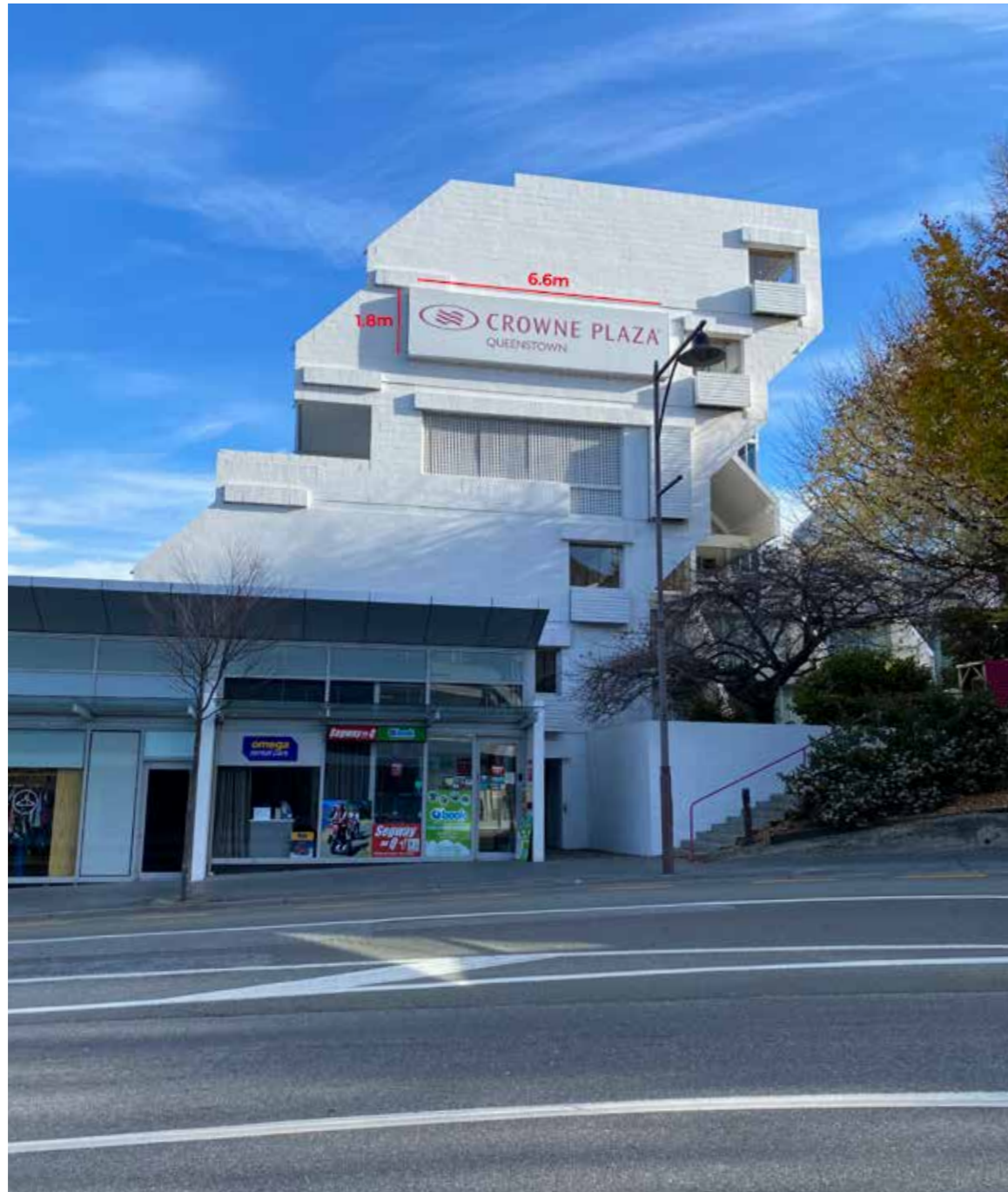
A. EXISTING VIEW OF THE NORTHEAST ELEVATION OF THE CROWNE PLAZA BUILDING
