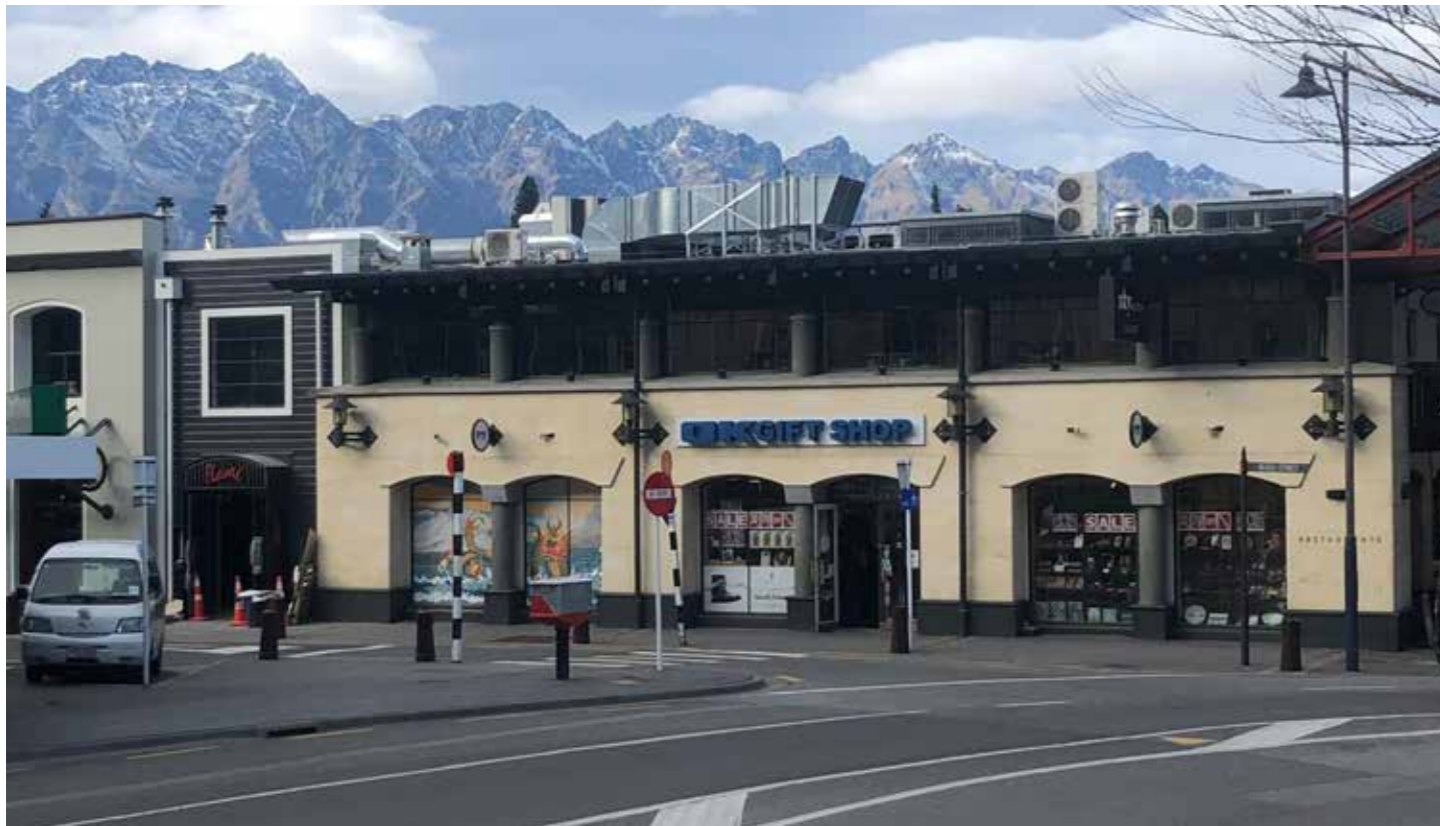
C View from the base of the billboard looking towards Steamer Wharf. Steamer wharf is a 2 storey development on the lakefront designed to appear as several independent buildings linked by internal, covered walkways. Building utilities are clearly visible on the building's roof.
