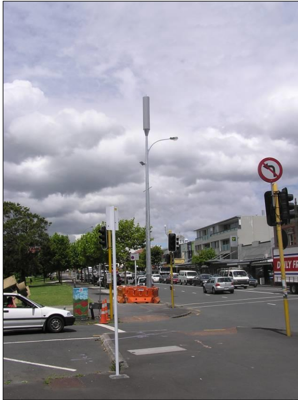
Figure 2: Typical Spark light pole on Ponsonby Road, Auckland (example is 15m high)
