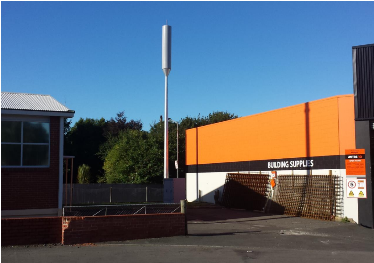
Figure 1: Vodafone mast at 18 Church Street, Mosgiel (example is 12m high)
