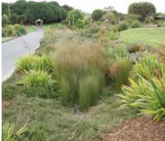
Figure 8 – Example vegetated swale
