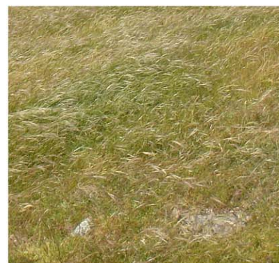
turf roof: vegetation & soil over concrete structure
