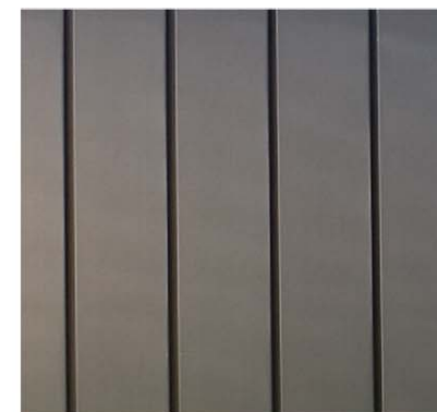
garage / storage // facility room door: preweathered zinc sheet over ply substructure
