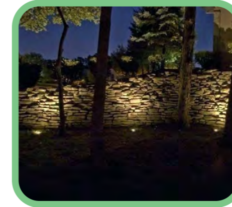
Feature uplighting To be directly focused towards features being illuminated, such as trees, buildings signs and stone walls in a way to minimise light spill. Fitting to be Hunza Lawn Light 6 Watts 3000k
