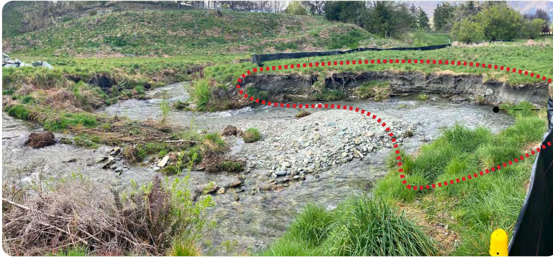
Before erosion protection
