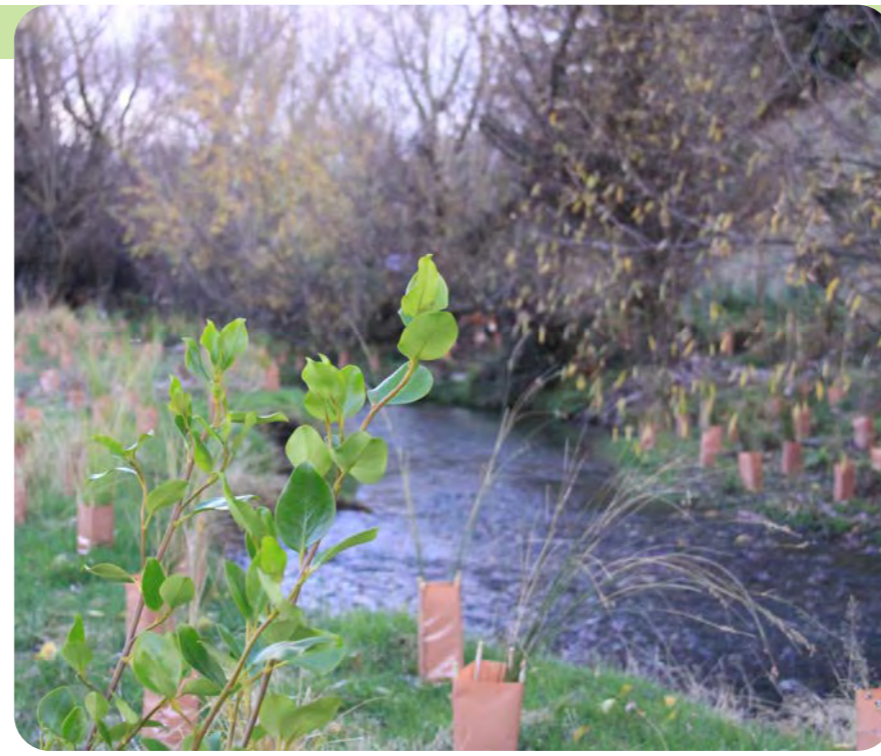
Riparian revegetation planting works underway along Mill Creek (within the applicants land)
