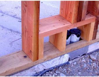
Untreated Douglas Fir used as framing. In this case treated Radiata is used for the bottom plate.
