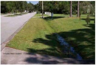
4)Infrastructure such as swales for storm-water and constructed wetlands for wastewater treatment can be landscaped to form features that can double as reservoirs for irrigation.
