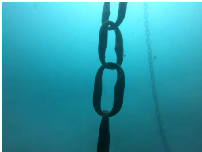
Underwater view of the mooring riser chain during the dive
