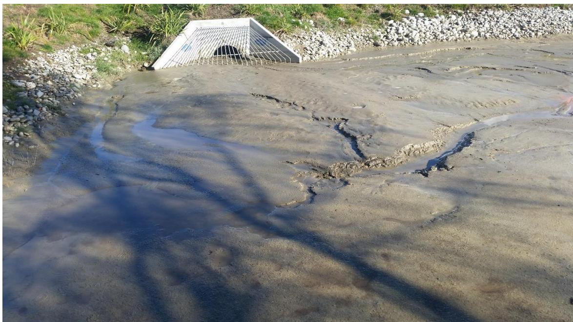
Figure 4: Heavy silt trapped in the sediment forebay stormwater retention dam upstream of Bullock Creek Hatchery Springs 3 days after the event on 22 May 2018.
