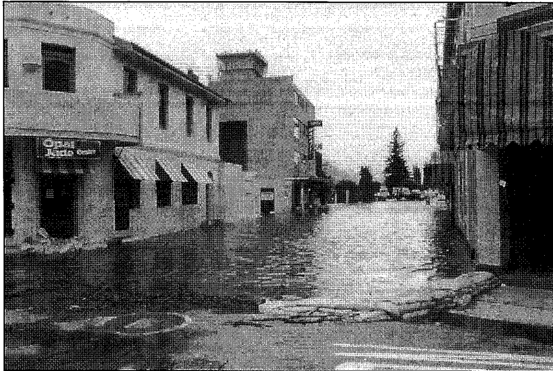
Photograph 5 Queenstown Flooding at Beach Street (15 January 1983)
