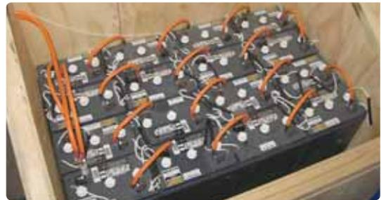
The batteries for this SAPS are well protected and secured in this box, preventing unauthorised access.
