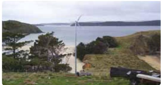
Self-supporting tubular tower mounted three-bladed horizontal-axis micro wind turbine.
