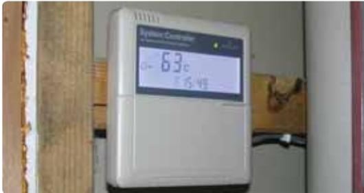
A typical controller for a solar water heating system.
