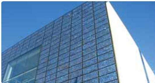
The façade of this building has integrated PV panels built into it.
