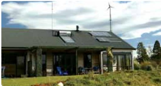
This photo shows a solar water heating system, solar photovoltaics, and micro wind turbine in a SAPS.
