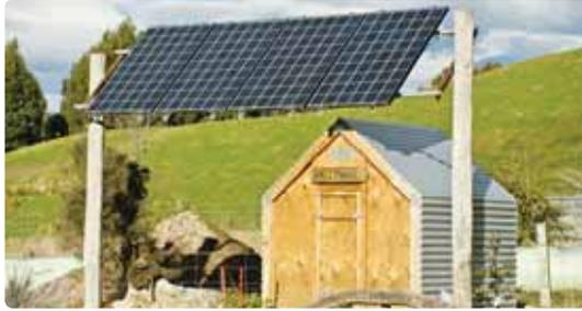
A ground mounted PV array in a SAPS.
