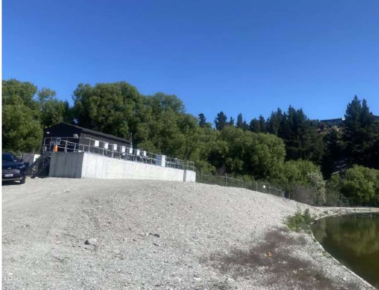
Figure 2 Current UV site at Shotover WWTP, photo taken 2024
