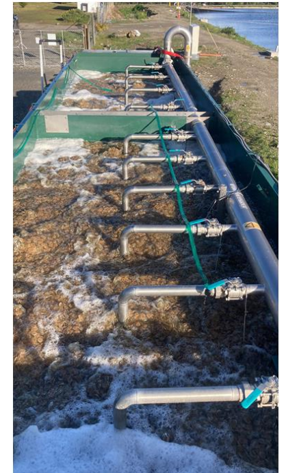
Fig 1. Moving Bed Biofilm Reactor at Hāwea WWTP
