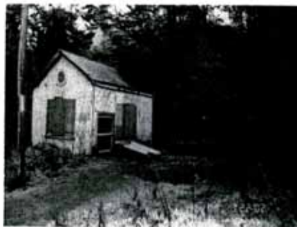
View from southern approach showing Powerhouse and adjoining concrete slab and upstand
