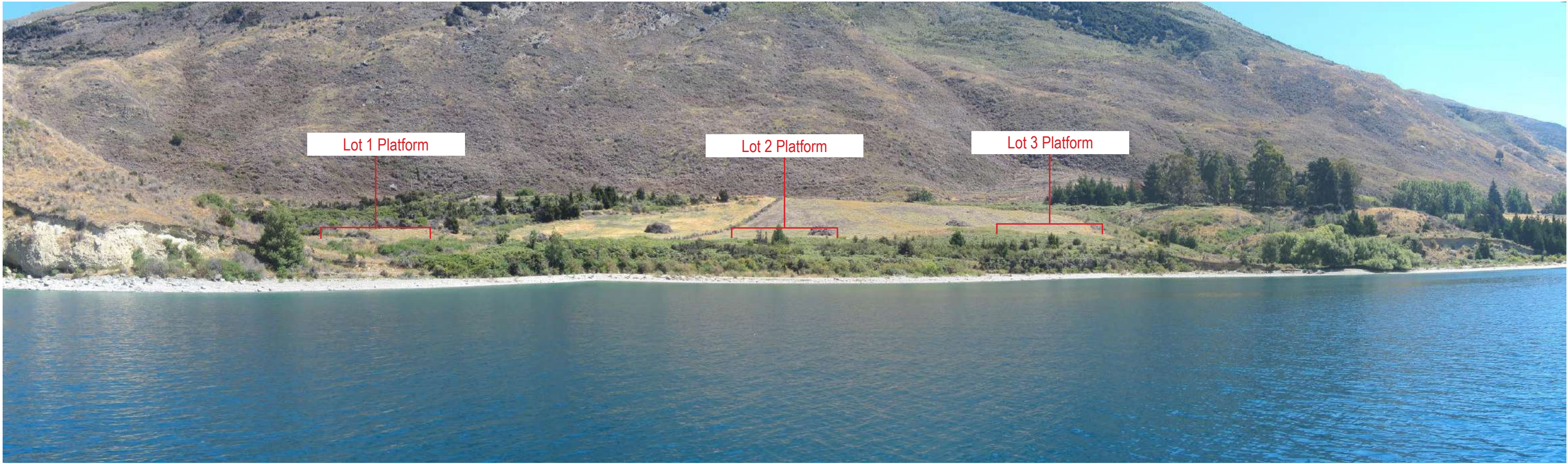
Viewpoint D - On the lake 200m from the boundary. Building profile poles have been used to depict approximate building envelopes in this image.
