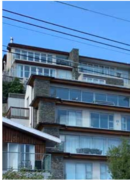
Apartment style units stepping up the hillside allow for greater development potential without breaching height controls
