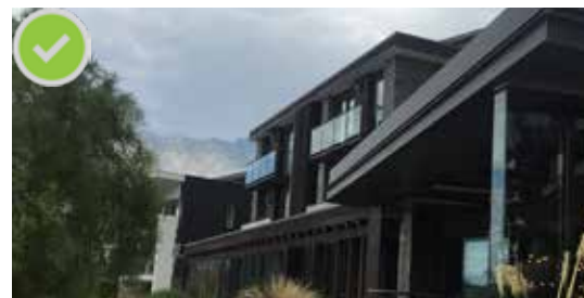
Planting can provide a soft buffer between private and public spaces without needing fencing.
