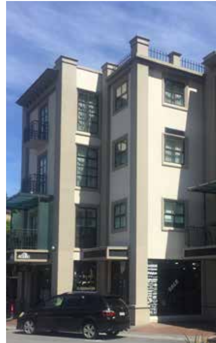
Four to five storey buildings are expected in the Queenstown BMU (note this is in the Queenstown Town Centre).
