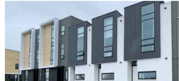
Terrace housing on sites less than 200m 2 is a common typology where shared facilities are not provided.
