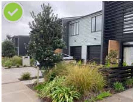
Linera board, steel and timber mix
