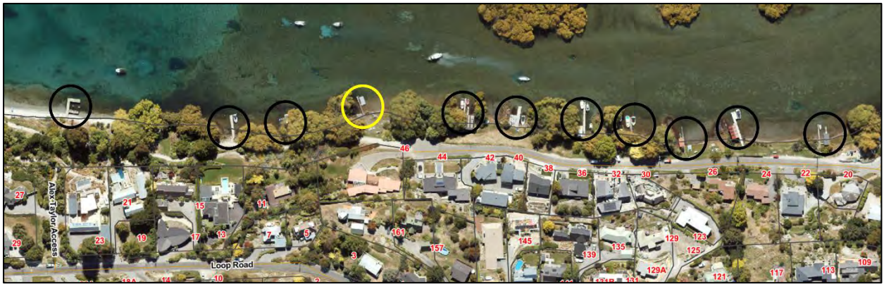
Figure 6: Receiving environment, Site circled in yellow and other boatshed/jetty structures shown in bold
