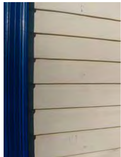
Timber weatherboard.
