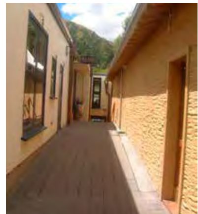
Uninteresting pedestrian link with poor detailing.
