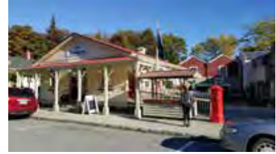
Open Space area to the north west side of Post Office, which is now integrated with the Post Office Precinct development to the rear.
