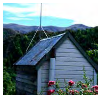
Shed, 18 Wiltshire Street.
