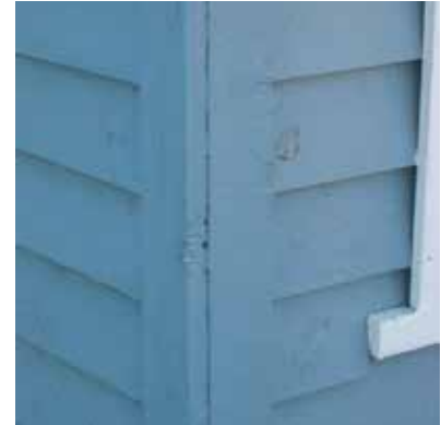
Painted Weatherboard with boxed corner.
