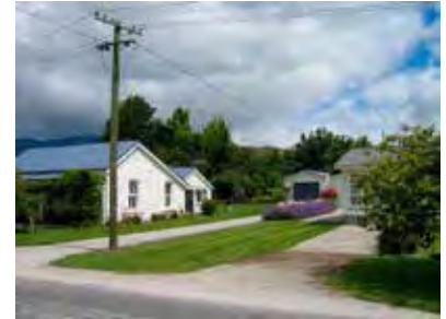
Garage set to rear of section.
