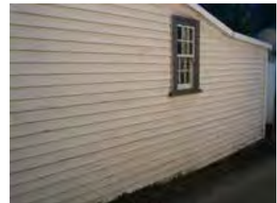
Painted Weatherboard with boxed corner.
