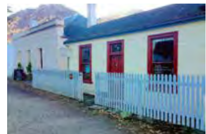
Good example of Picket fencing outside Miner's Cottage, Buckingham Street.
