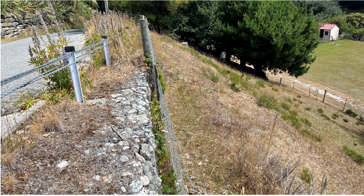
Figure 2: Photo of Atley Road, south of Mathias Terrace showing western boundary of existing carriageway
