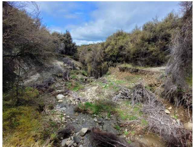
Figure 5-6 Main erosion basin / drop, looking downstream
