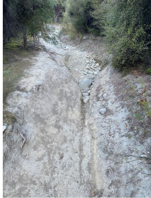
Figure 5-4 Adjacent to upper gully - erosion of mountain bike track
