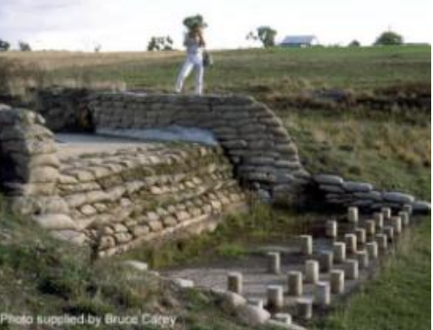
Sandbag drop structure (NSW)
