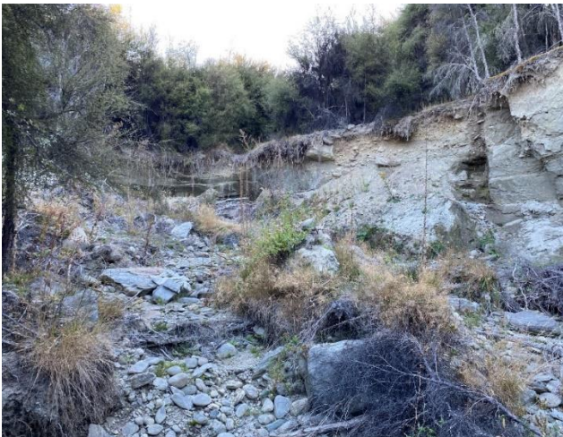
Figure 5-5 Main erosion basin / drop, looking upstream
