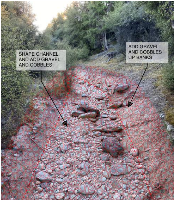
Figure 8-3 Sketch of example of area where channel would be shaped and rounded gravel and cobbles added to provide more natural mobile waterway bed.
