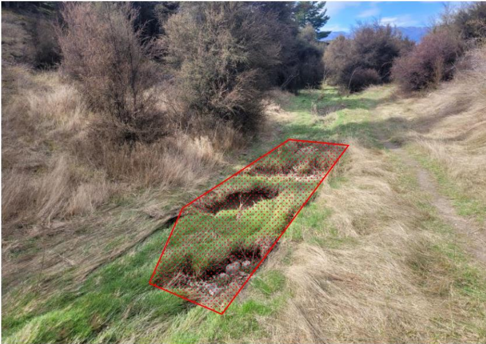
Figure 8-2 Sketch of example of area of existing erosion to be filled and re-grassed.
