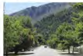
Casseron Street looking west, showing narrow carriageway, gravel shoulders and grass-verges and established street plantings, all of which are characteristic of the ARHMZ.
