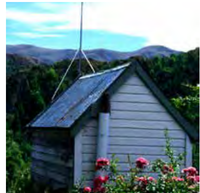
Small shed-out building.
