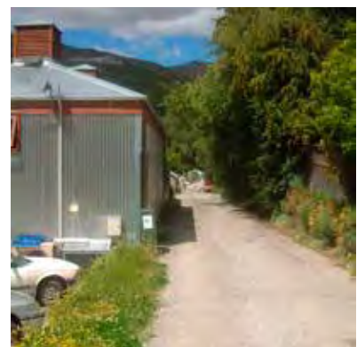
Arrow Lane, building (left) intrudes on the lane.
