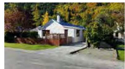
Dwelling located on Nairn Street, reflecting smaller scale Arrowtown properties found throughout the ARHMZ.
