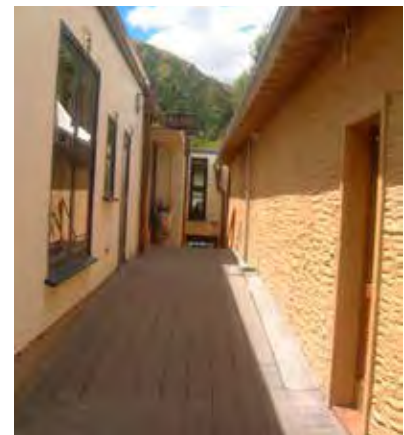
Uninteresting pedestrian link with poor detailing.
