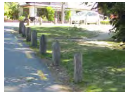
Good example of simple timber bollard.
