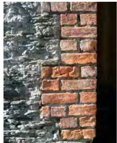
Brick used sparingly.
