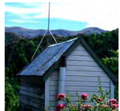
Shed, 18 Wiltshire Street.
