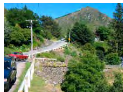
Butlers wall, Villiers Street behind.
