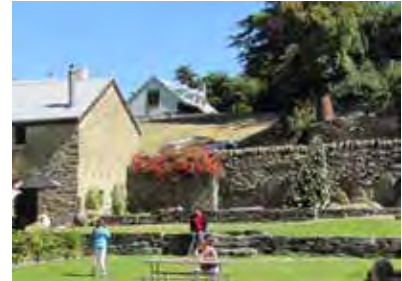
Looking east towards Arrow Lane from the Buckingham Green, showing existing residential dwelling located within Neighbourhood 1 – Above Town Centre.
