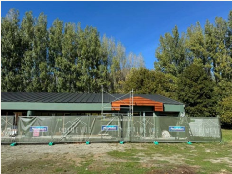
516 Ladies Mile – Exterior Upgrade
