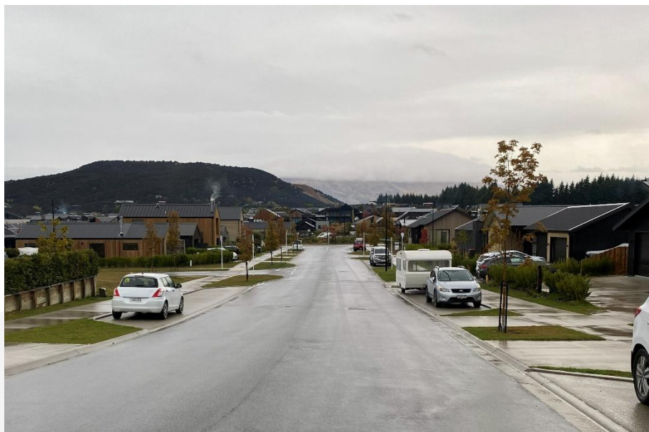
Photograph 6: Typical Cross Section of Riverslea Road
