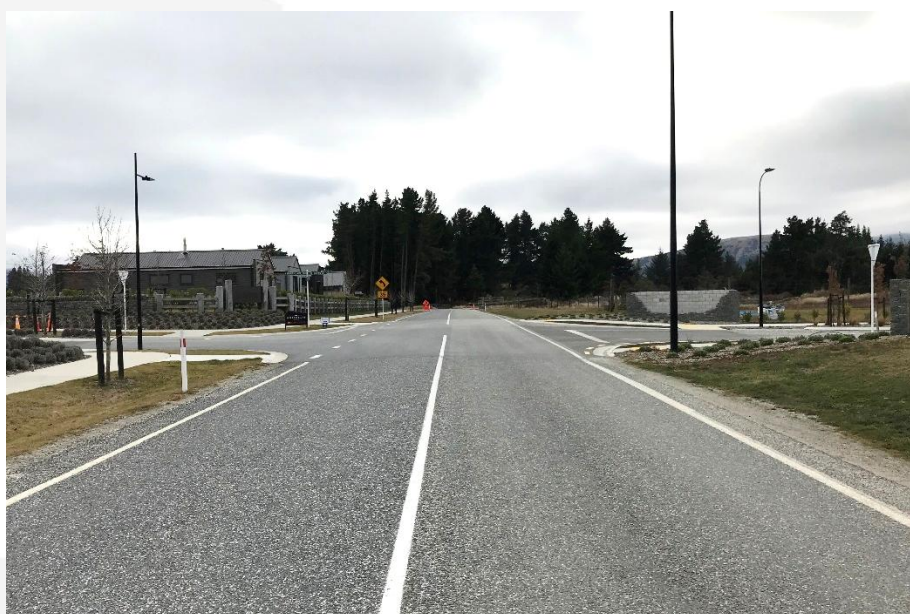
Photograph 10: Outlet Drive Looking North, Northlake Drive on Left
