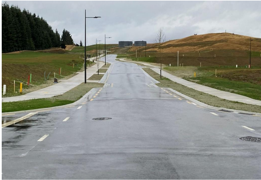
Photograph 3: Northern Section of Stonehenge Road (Looking North)
