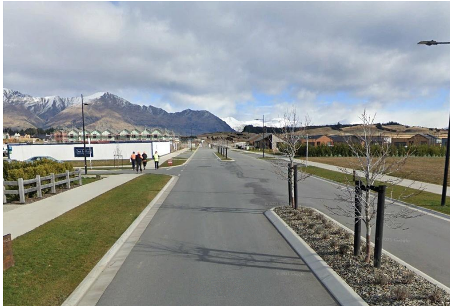
Photograph 9: Northlake Drive (Looking West)
