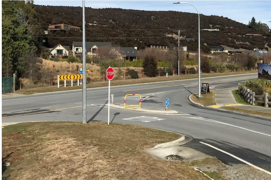
Photograph 11: Aubrey Road / Outlet Road Intersection
