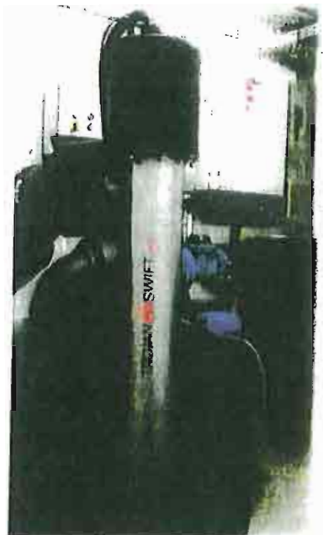
The compact Trojan UVSwift™ SC system can easily be accommodated in very restrictive spaces, and can be mounted vertically or horizontally. Shown with optional automatic wiping system.
